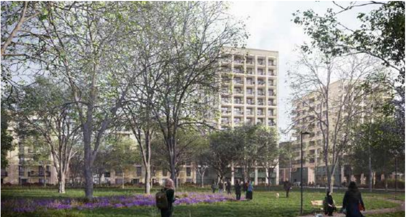
The new council homes to be built at the Ashley Road Depot site, looking north from Down Lane Park
