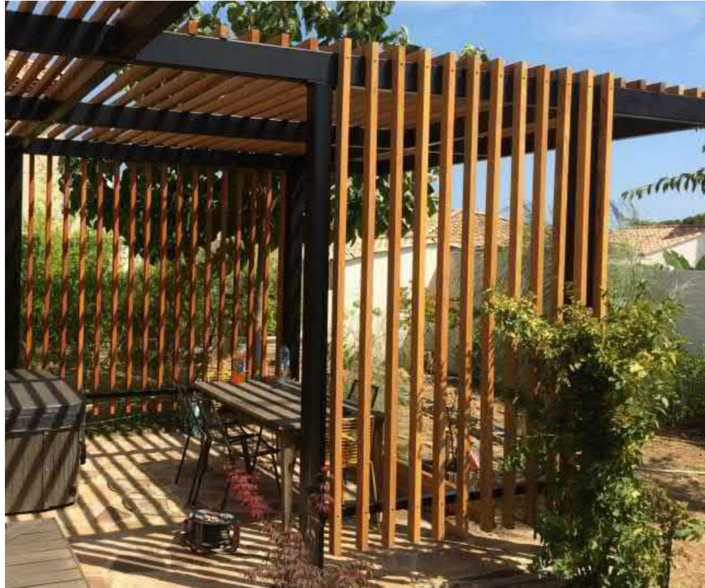
Timber pergola with in-filled roof/walls
