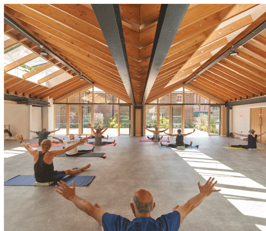
Double height internal spaces with exposed timber frame structure
