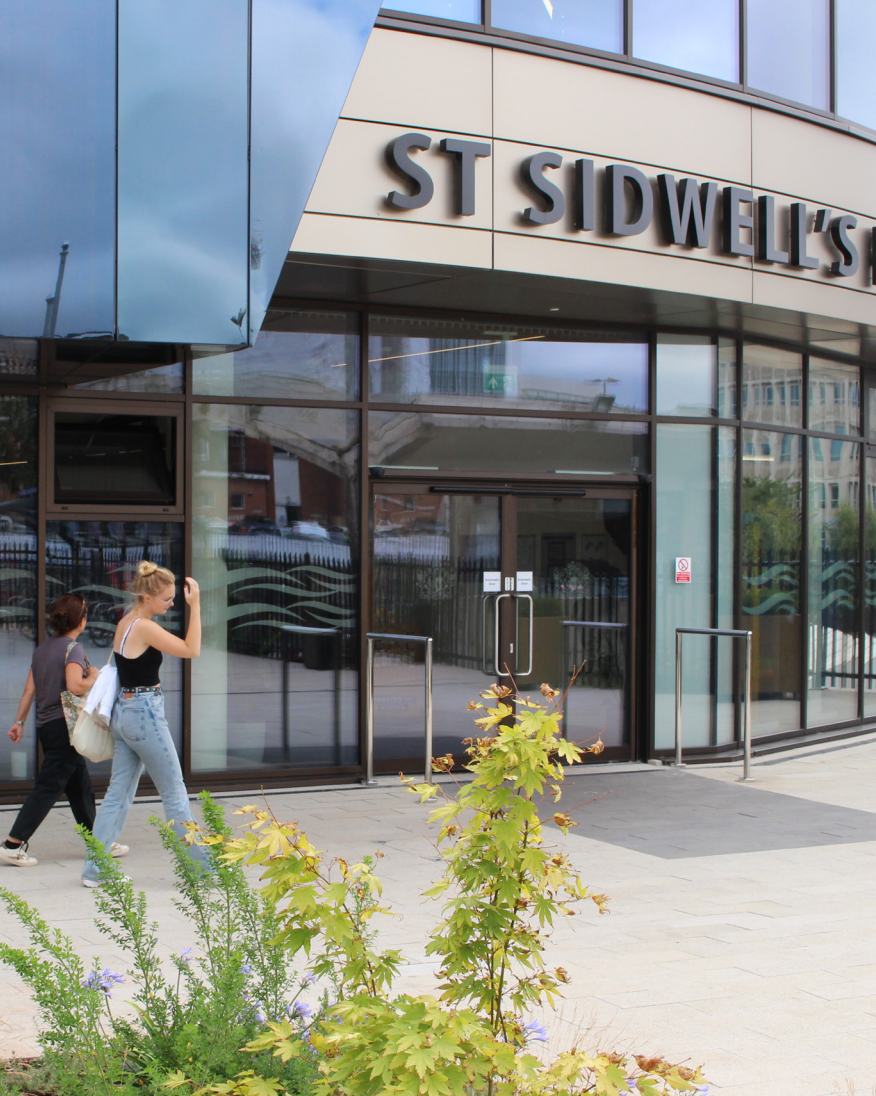
St Sidwell's Point is the UK's first Passivhaus pool demonstrating the City's commitment to leading the way in net zero carbon, promoting innovation and placing Exeter on the global stage
