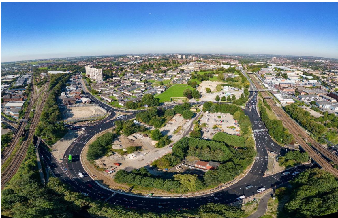
Aerial photo indicating the progress made at the Armley Gyratory Project
