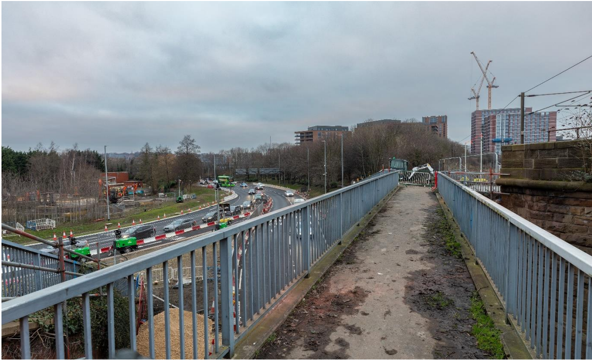
First installed in 1970, the old bridge was 1.8 metres wide.
