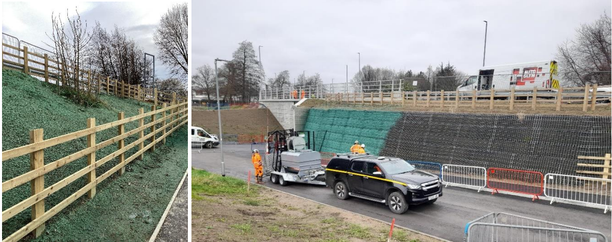
The earth retaining wall at Armley Gyratory
