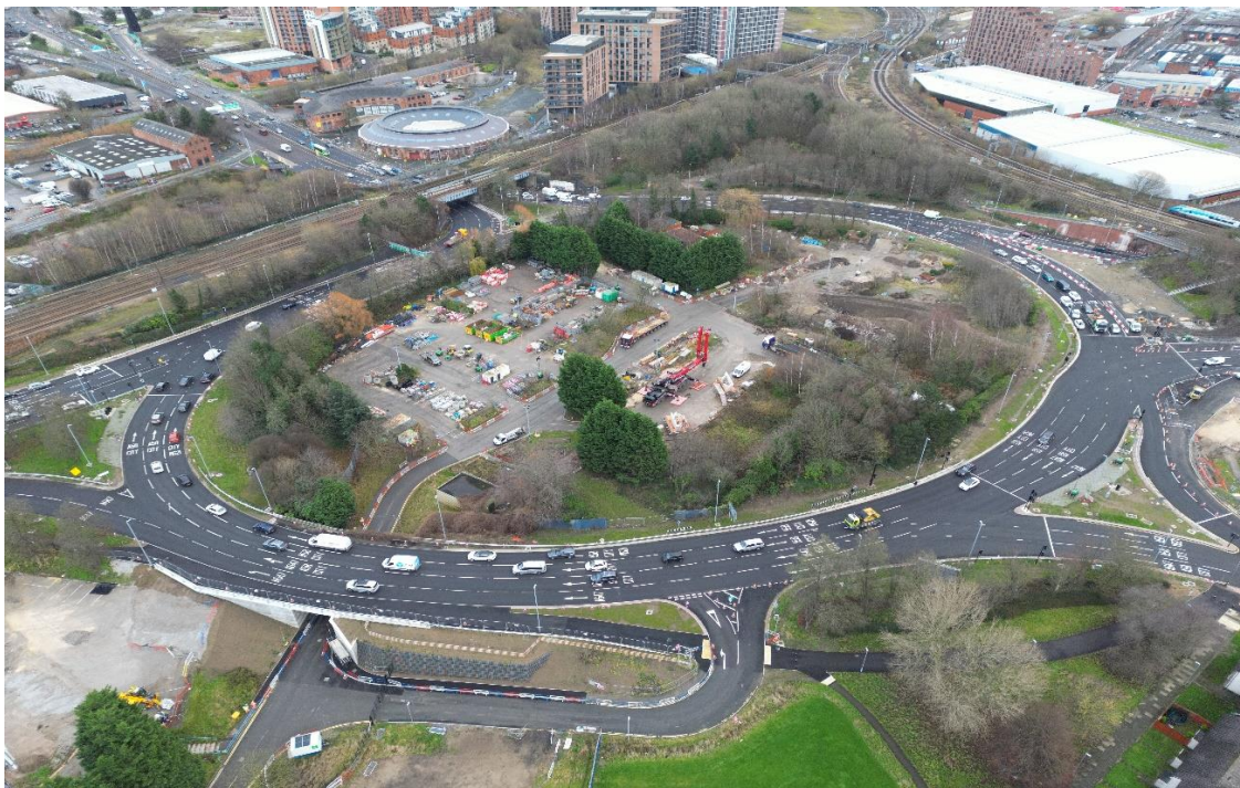
January 2024- Armley Gyratory looking east towards Leeds City Centre, prior to the Gelderd Road footbridge replacement.
