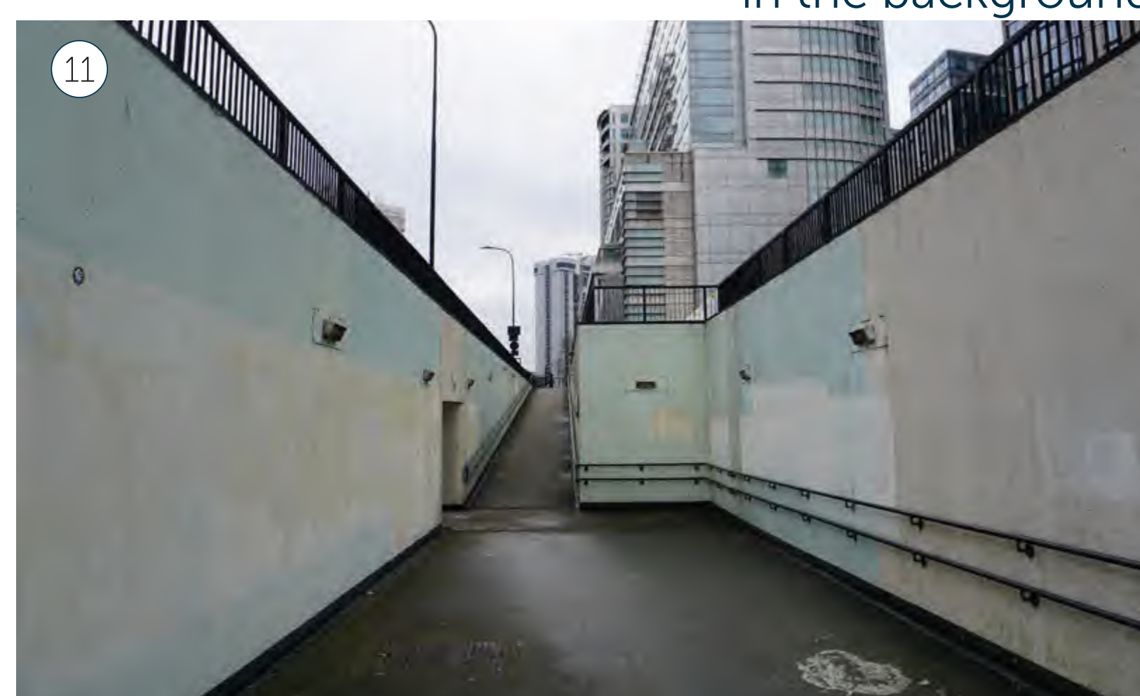
Existing: Westway Underpass southern entrance
