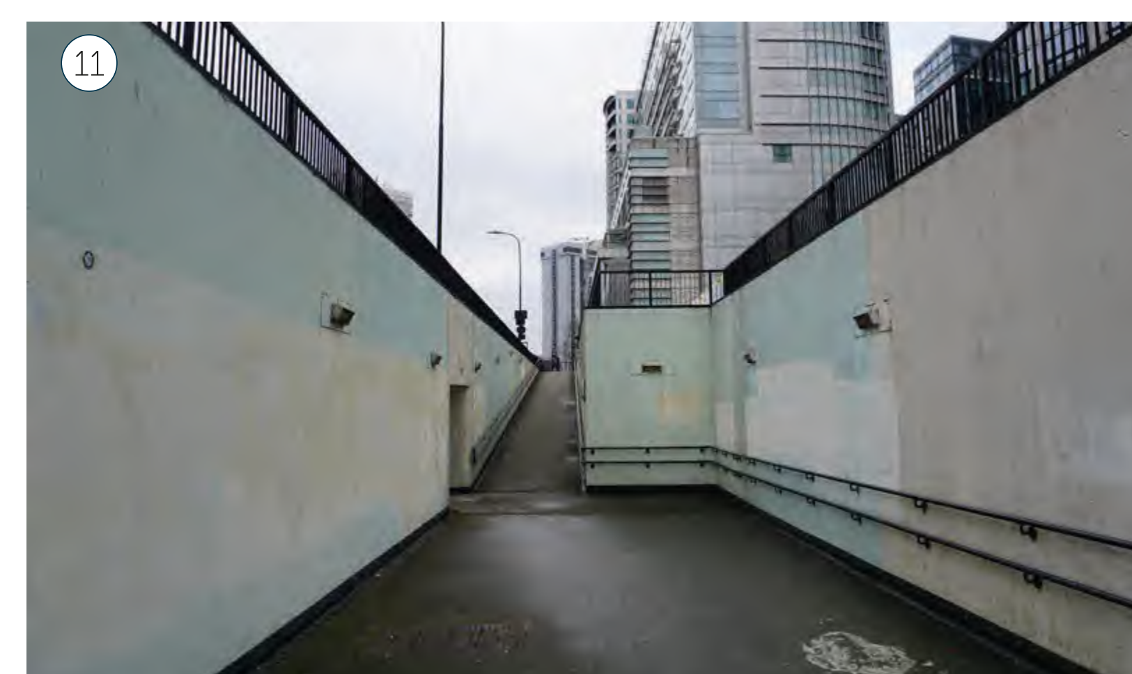
Existing: Westway Underpass southern entrance
