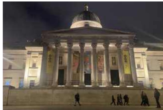
National Gallery Lighting of historic building and evening activity
