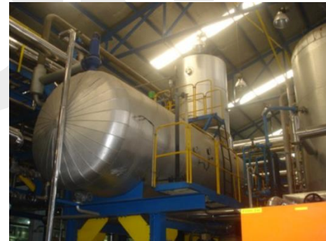
Condensate water recovery pipe connected to boiler feed water tank
