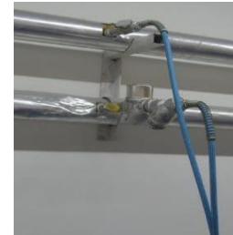
Picture of a condensate pipe for ironing process with a steam trap on condensate pipe
