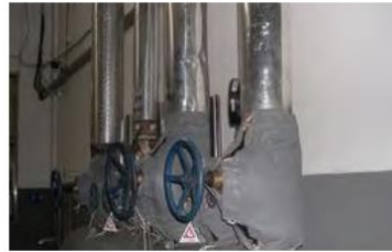
Various insulation jacket configurations over valves
