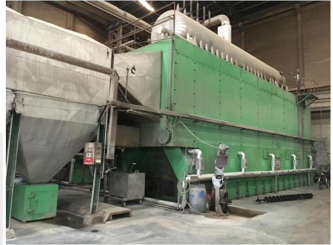
Biomass boiler in dye mill
