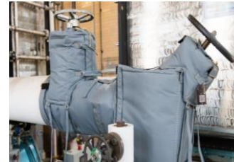
Various insulation jacket configurations over valves
