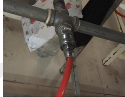
Compressed air pipe connection point to be checked for leak
