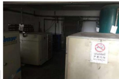
Insufficient ventilation in compressor room
