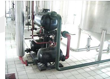
Condensate collection unit and pipework pumping condensate to centralized collection tank
