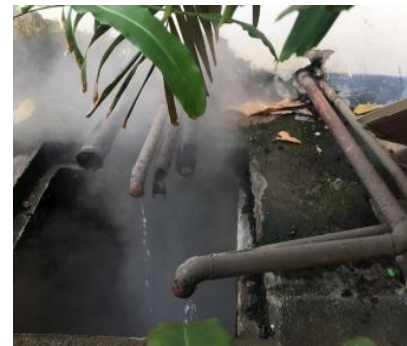
Example of apparel tier 1 facility discharging condensate water
