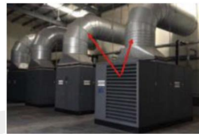
Compressors with hot air ducted outside
