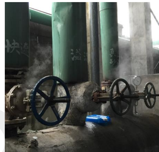
Steam leakage
