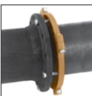
Insert the next bolt or stub opposite the first and again thread the nut on hand tight. Continue this procedure until all bolt holes have been fitted. Insertion of the flange bolts prior to contact of the flanges will help in the alignment of the flanges. Pull the two flanges into contact using care to assure that the gasket remains fully seated within the gasket cavity during assembly.
