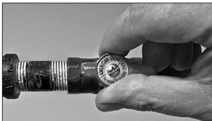
Figure 31 - Manual Gas Valve in ON position.
