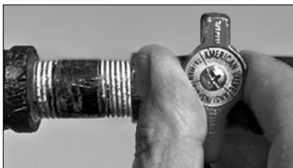
Figure 45 - Manual Gas Valve in OFF position.
