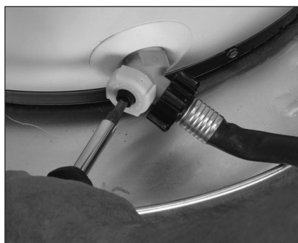
Figure 20 - Draining the old water heater.
