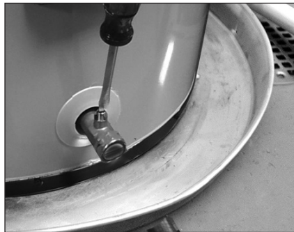
Figure 39 - Draining the water heater.
