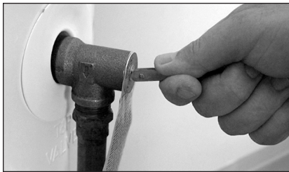
Figure 42 - T&P Relief Valve
