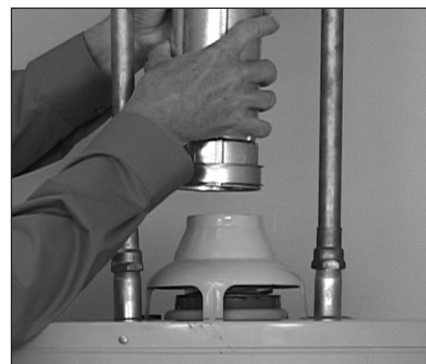
Figure 22 - Disconnect the vent pipe from the draft hood.
