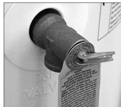
Figure 24 - Temperature and Pressure Relief Valve
