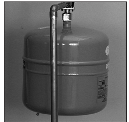
Figure 13 - A Thermal Expansion Tank helps protect the home's plumbing system from pressure spikes.
