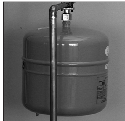
Figure 28 - The Thermal Expansion Tank should be pressurized with air to match the home's incoming water pressure.
