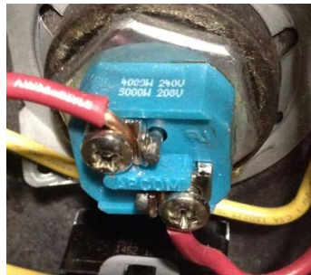
Figure 13. Example of Wattage/Voltage Marking on Element
