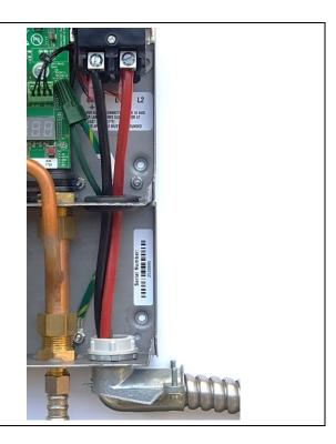
**2.** The power leads are to be secured to the L1 and L2 or L and N connectors on the terminal block or relay. The ground lead is to be secured to the GND connector on the block or the green ground wire with the provided wire nut.
