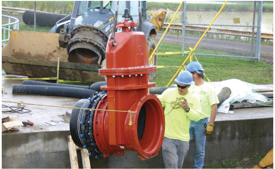
Installation of 24" Resilient Wedge Gate Valve
