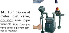
do not use pipe wrench. Note: Open gas valve slowly to prevent damage to regulator.
