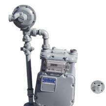
6. With original plumbing removed, build new plumbing from structure to meter.
