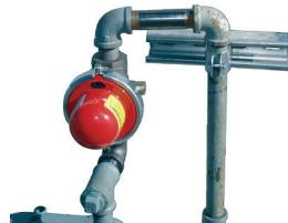
12. Finish meter plumbing system with PSP seismic valve.
