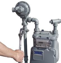
2. Turn gas off at meter inlet valve, **do not** use a pipe wrench.
