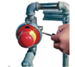
14. Turn gas on at meter inlet valve, **do not** use pipe wrench. Note: Open gas valve slowly to prevent damage to regulator.
