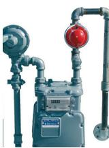
9. Install union gasket and new plumbing from meter to building.
