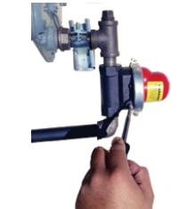
13. **While gas is still off**, open seismic valve. **Do not** open against gas pressure.
