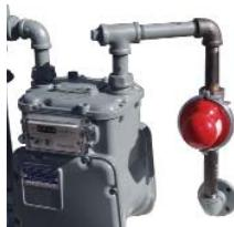
9. Install union gasket and new plumbing from meter to building.
