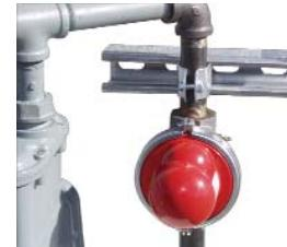
11. Install stabilizer bracket ( Unistrut or equivalent ) to plumbing ( within 6" of valve ) and secure to building.
