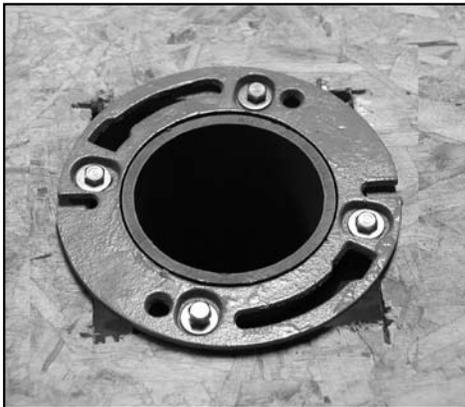
In the majority of installations too much wood has been removed to properly secure a round closet flange.
