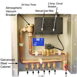
Special Calibrated Manifold for Equal Water Distribution to Floor Drains
