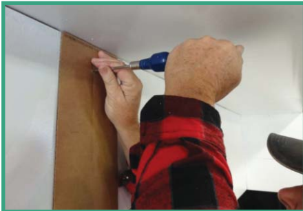
Using the template mark the hole locations
