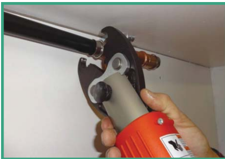
Make the Viegas PEX connection
