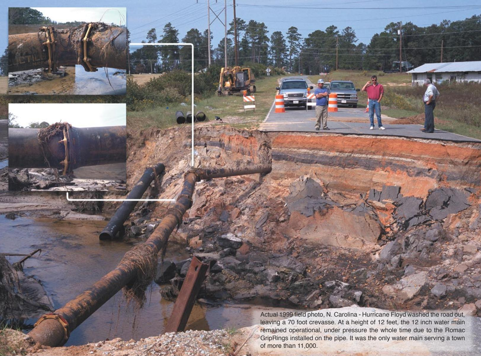
Actual 1999 field photo, N. Carolina - Hurricane Floyd washed the road out, leaving a 70 foot crevasse. At a height of 12 feet, the 12 inch water main remained operational, under pressure the whole time due to the Romac GripRings installed on the pipe. It was the only water main serving a town of more than 11,000.
