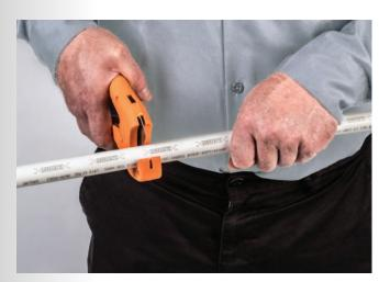
**Step 1**Cut the desired length of pipe.
