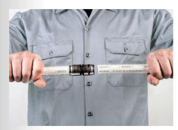
**Step 3**Push the pipe into the fitting firmly.
