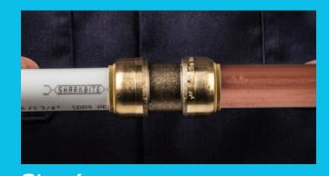
Step 4 Push the tubing into the fitting.
