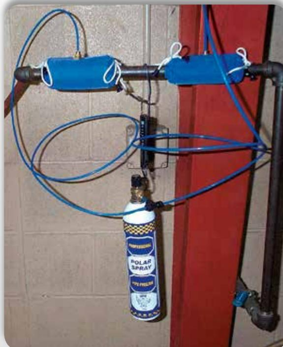
Wheeler's Pipe Freeze Kits install in seconds on pipes up to  $2\frac{3}{8}$ " O.D. and require no special tools. Ice plugs last 15–20 minutes and can be easily renewed.
