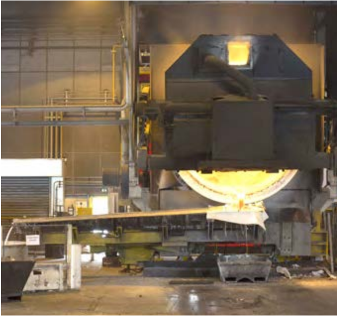
▲ Casthouse furnace at our site in Neuf-Brisach
