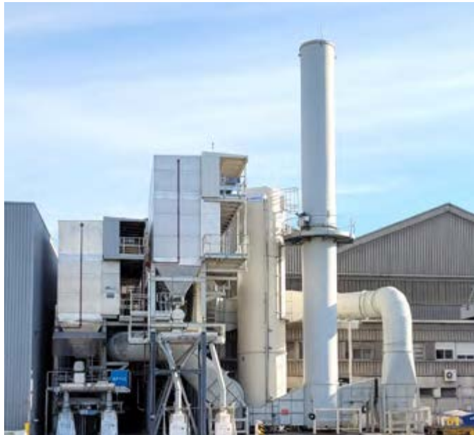
▲ Recently installed air filtering device at Issoire
