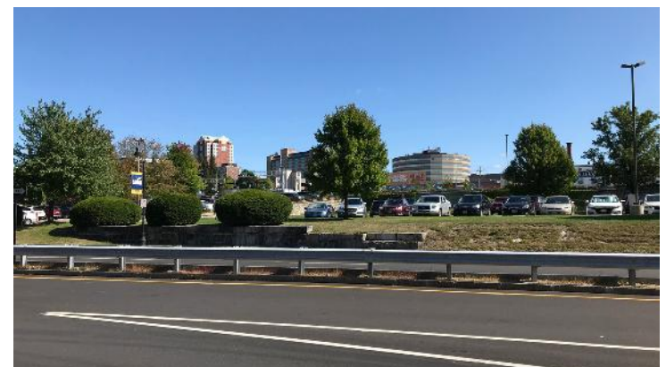
Significant grade changes and restricted pedestrian access make it difficult to traverse many parts of the TOD area on foot, including S. Commercial Street.
