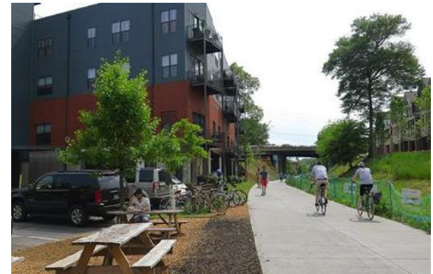
Site plans should orient towards pedestrian- and bike-friendly spaces and amenities like the Riverwalk and future rail trail. There should be clear visual and physical connections between these spaces and future development.
