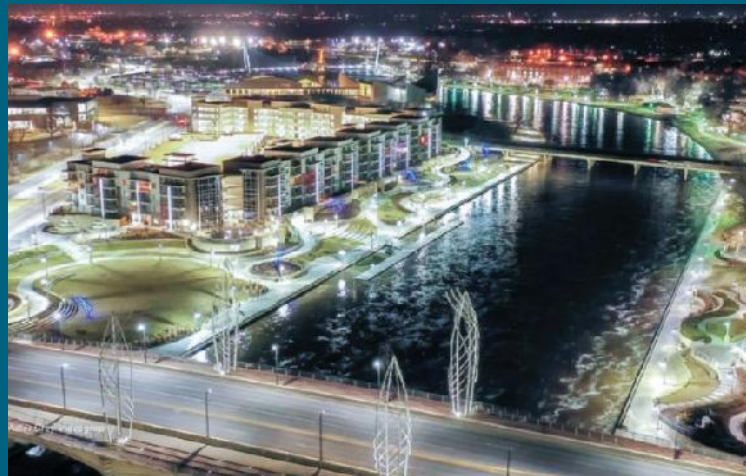
The City sold surplus riverfront land to a developer in return for reconstruction of a public park and riverwalk, and the 202-unit RiverVista housing development. The building includes a new boat storage and docks for Wichita State University rowing at river level.
