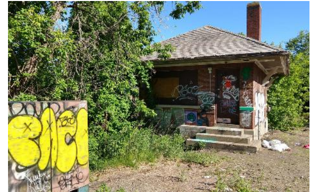
Currently abandoned, the historic Manchester Switch Tower will be at the heart of the new Switchyard District and future passenger rail station. Restoring the structure and providing public amenity space around it will make the Switch Tower a landmark of the district.
