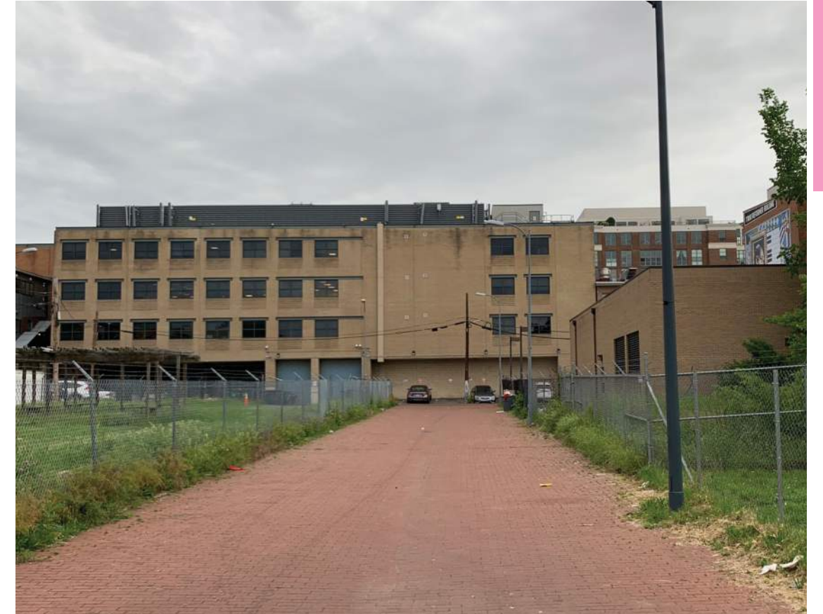
3. Existing Building South Facade - Temperance Ave, NW
