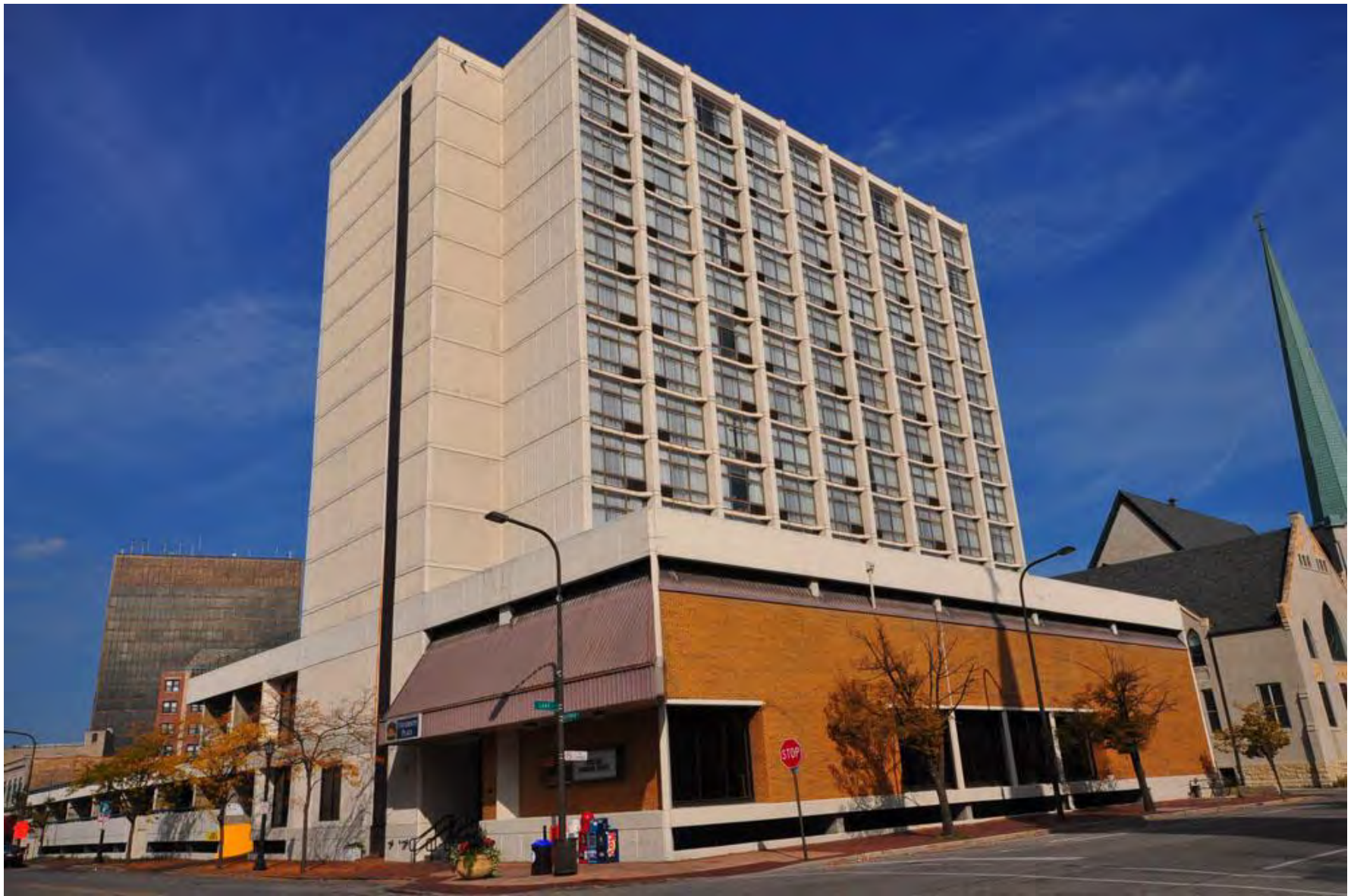
Holiday Inn – Northeast Corner Sherman Avenue & Lake Street
