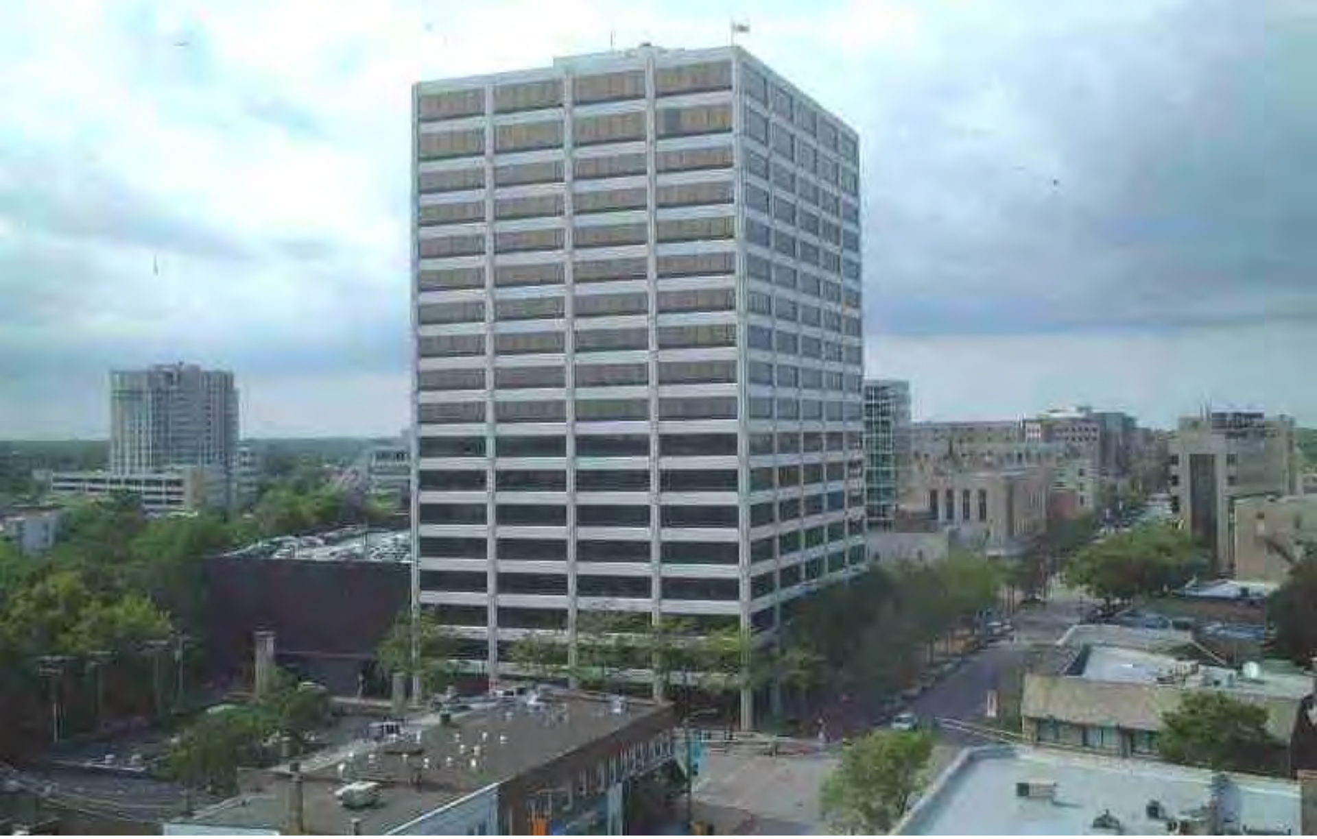
Rotary Building – Northwest Corner of Sherman Avenue & Grove Street
