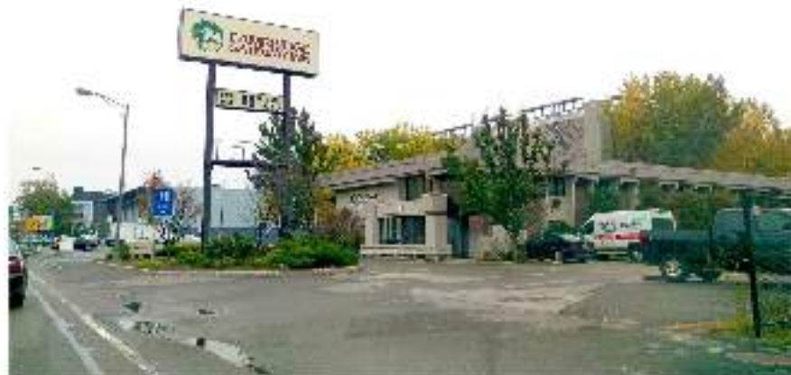
EXISTING INN ON PROPERTY - TO BE DEMOLISHED
