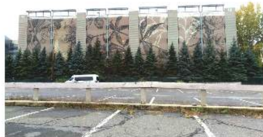
EXISTING PARKING GARAGE - BEHIND THE PROPOSED DEVELOPMENT
