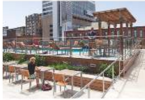
Raised Pool Deck
