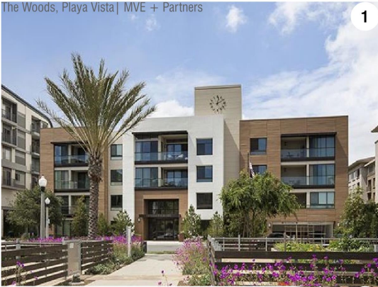
The Woods, Playa Vista | MVE + Partners
