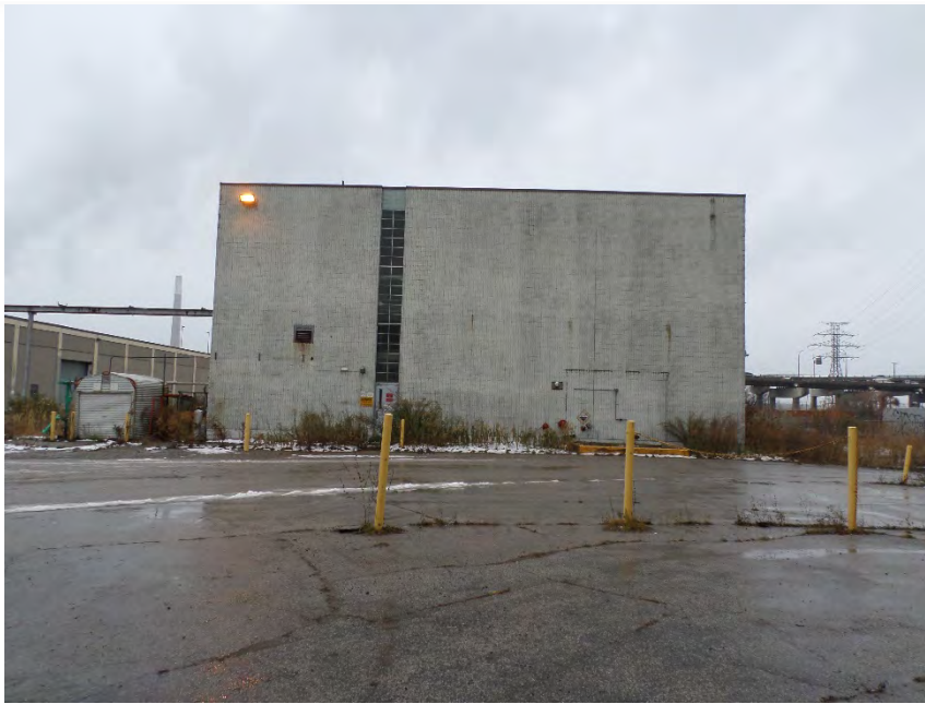
Photo 13 – View of Building 42, facing south.
