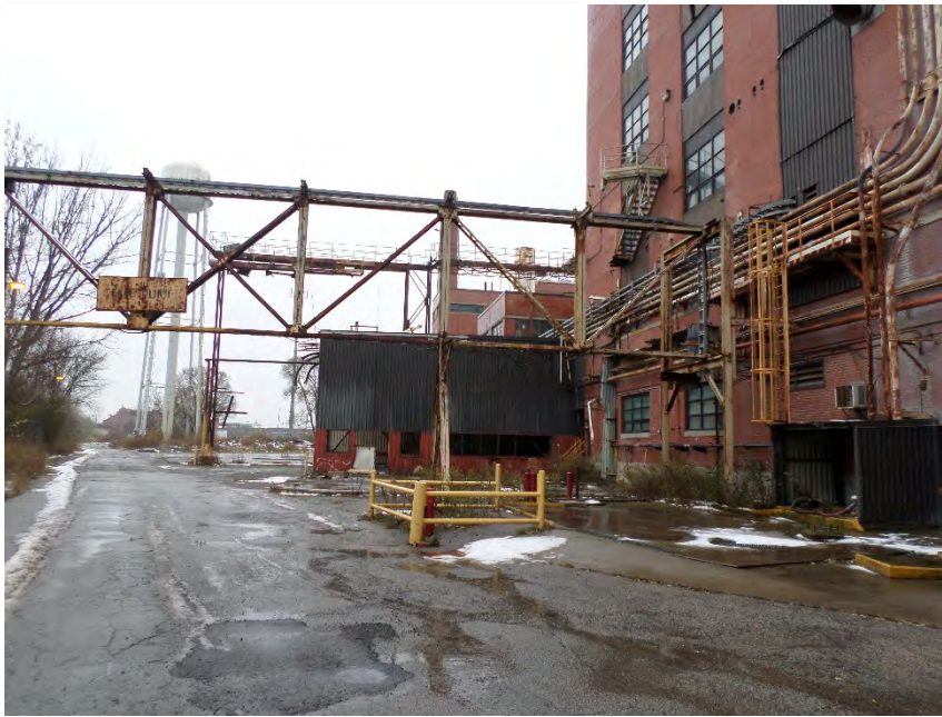
Photo 7 – View of the former tank and containment area located immediately north of Building 36, facing east.
