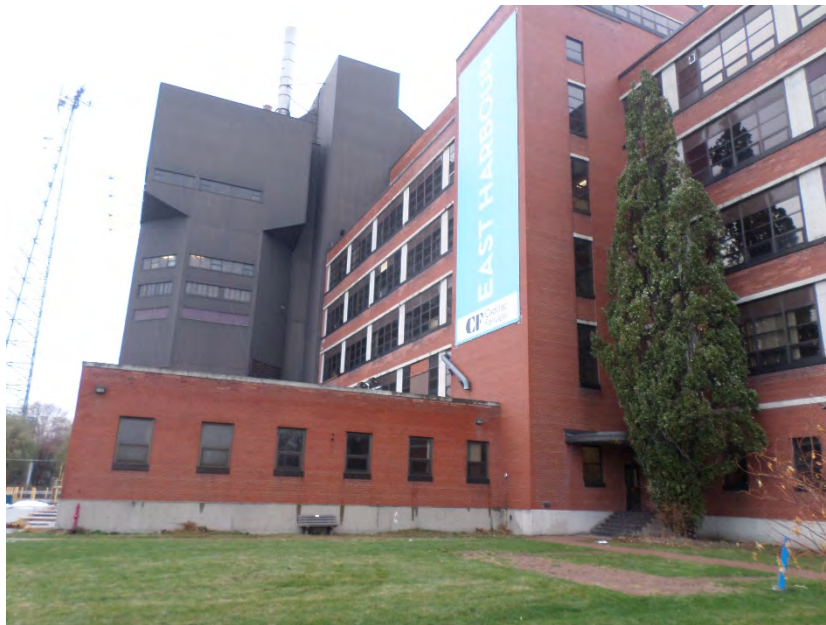
Photo 2 – View of west side of Building 36, facing north.
