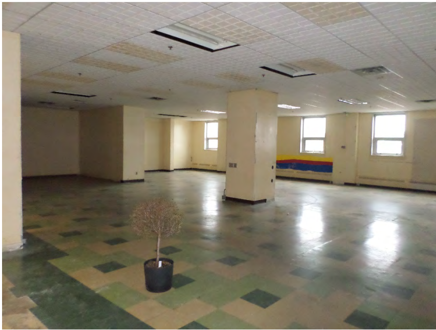
Photo 3 – Interior view of the ground floor area of Building 36.
