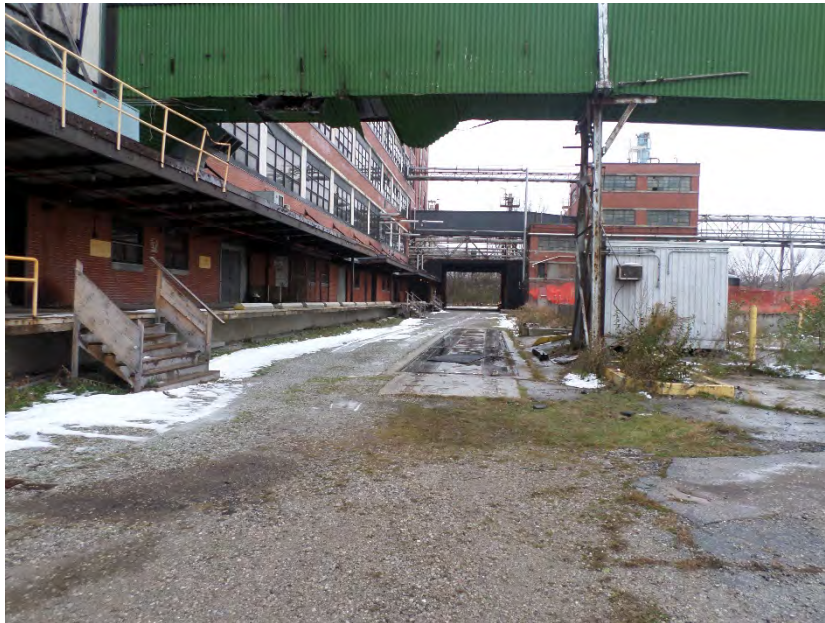
Photo 8 – View of the former rail spur area, between Building 36 (left) and Building 35 (right), facing north.
