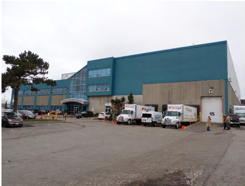
Photo 26 – View of the building at 30 Booth Avenue (facing west).
