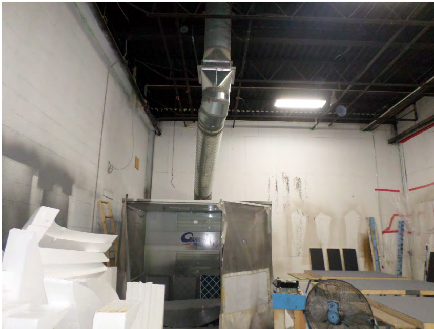
Photo 29 – View of paint booth within the building at 30 Booth Avenue, used for painting film sets.
