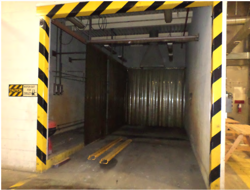
Photo 19 – View of former forklift wash area with location of out-of-use oil water separator (Building 41).
