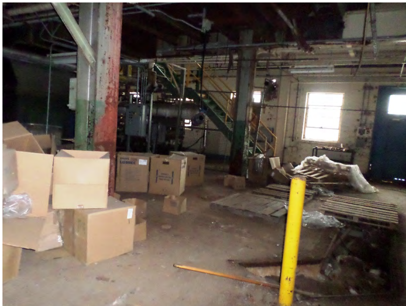
Photo 12 – Interior view of the former Boiler House (Building 38).
