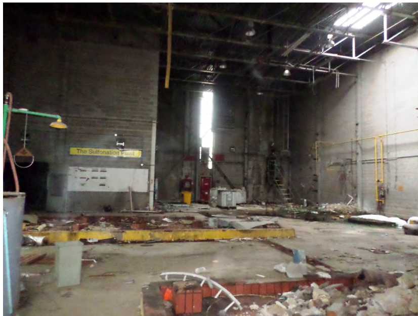
Photo 14 – Interior view of Building 42, former Chemithon / Sulphonation Plant).
