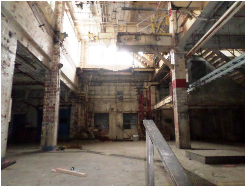
Photo 9 – Interior view of Building 35, former Liquids Building.
