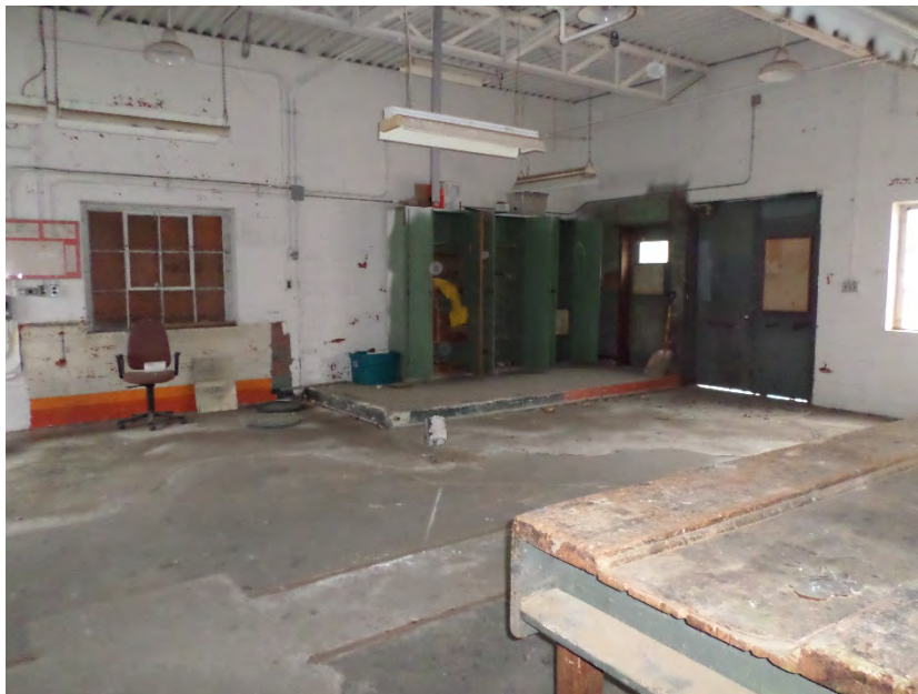
Photo 16 – Interior view of the former Carpenter Shop (Building 40).
