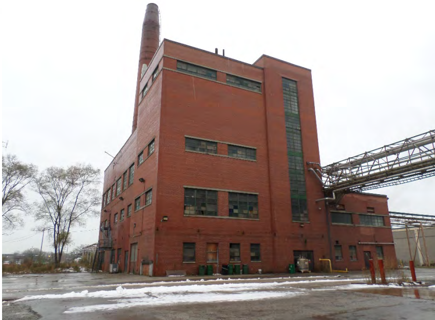
Photo 11 – View of the former Boiler House (Building 38), facing southeast.
