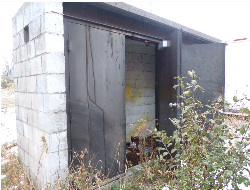
Photo 15 – View of self-contained former chemical storage shed.
