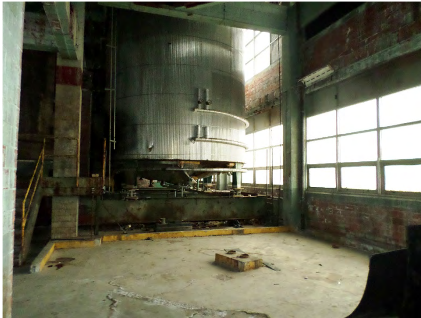
Photo 4 – Interior view of former manufacturing area on the sixth floor of Building 36.
