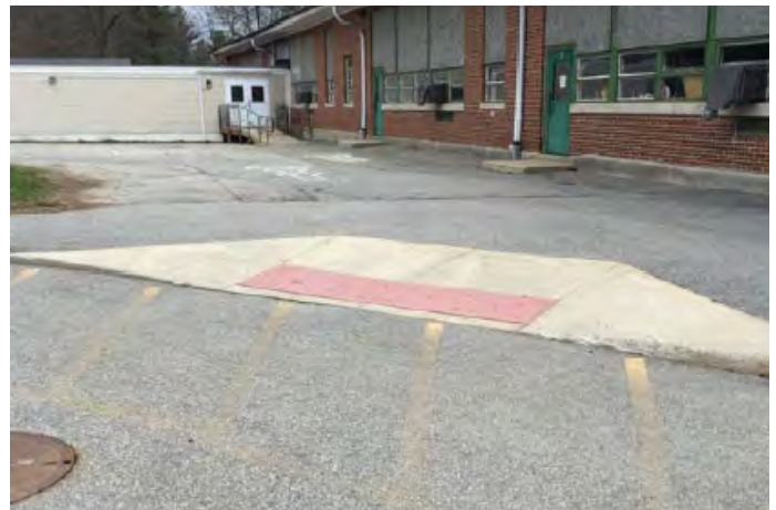
Drop-off at parking loop leading to modular classrooms doorway
