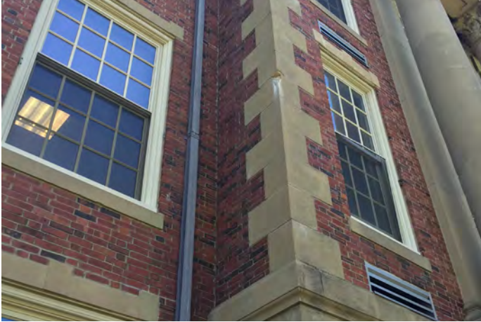
Brick at exterior of building
