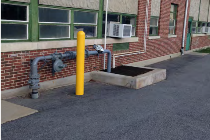
Recently repaved parking lot
