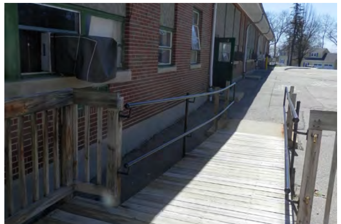
Handicap accessibility ramp
