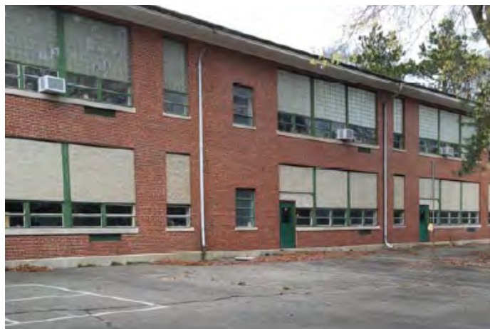
Abandoned lower courtyard
