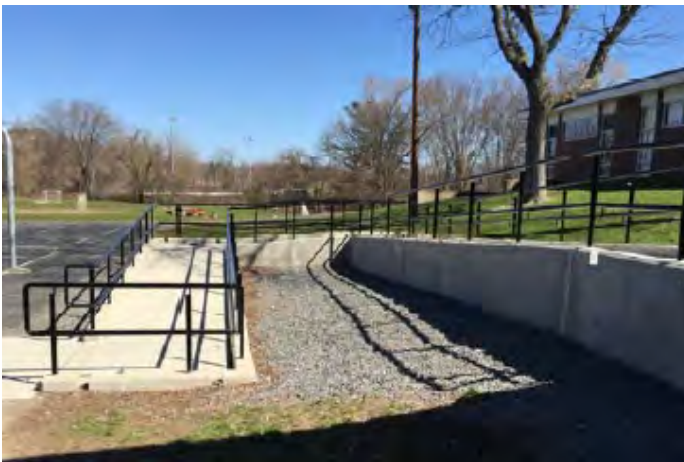
Service to athletic courts off Tufts Road
