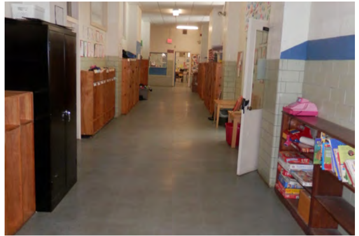
Typical flooring in hallway
