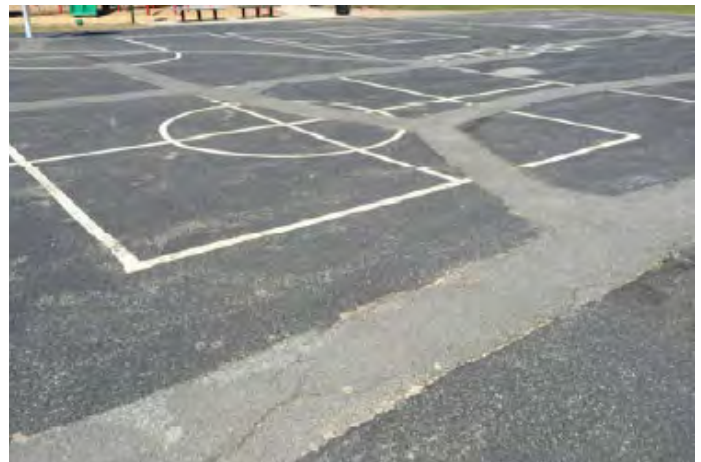
Extensive crack repair at basketball court pavement
