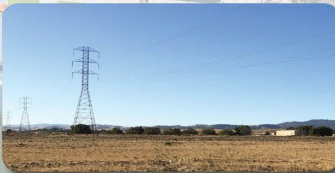
Overhead electrical lines
