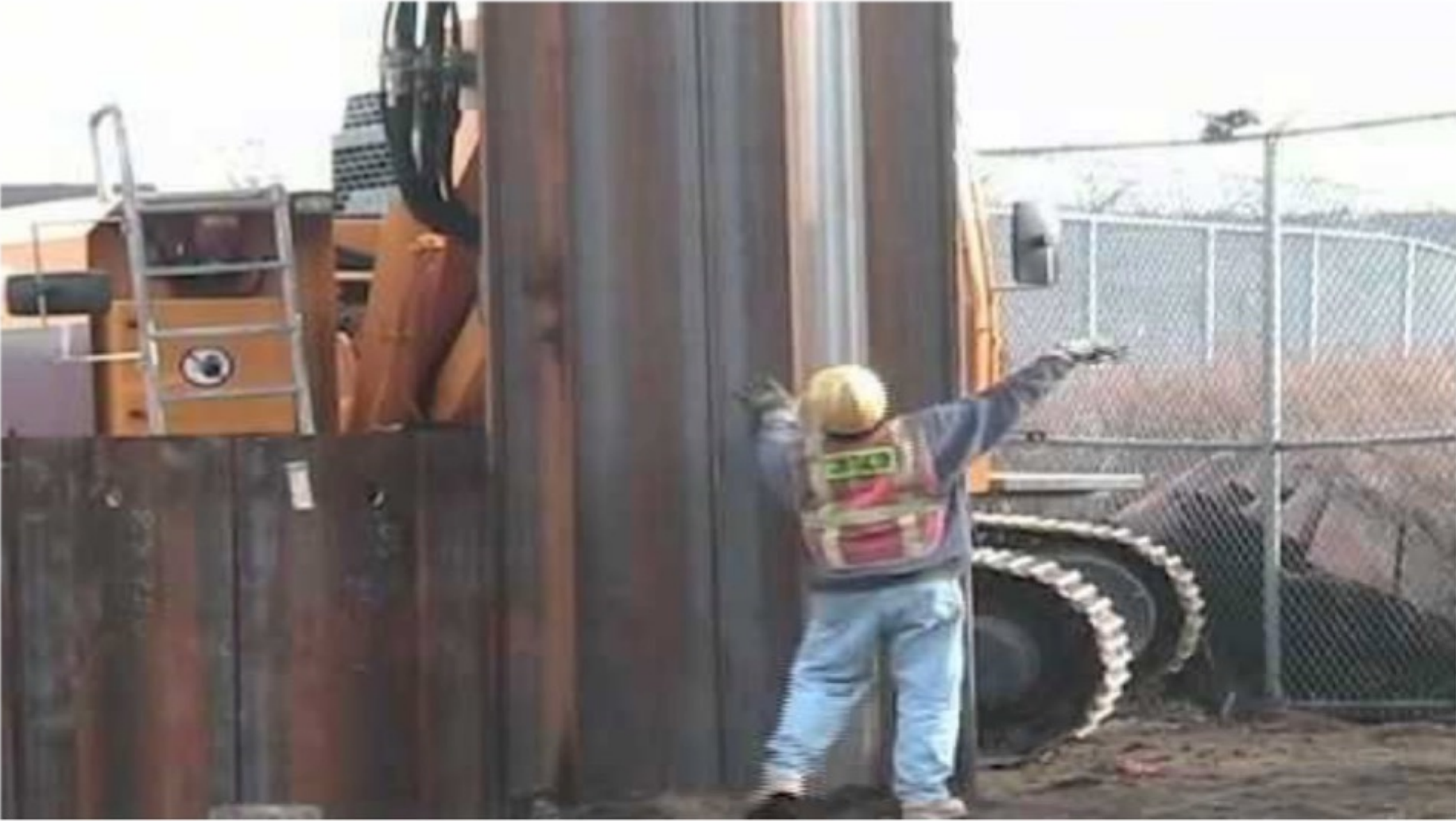
Click on Image for Video of Sheet Piling
