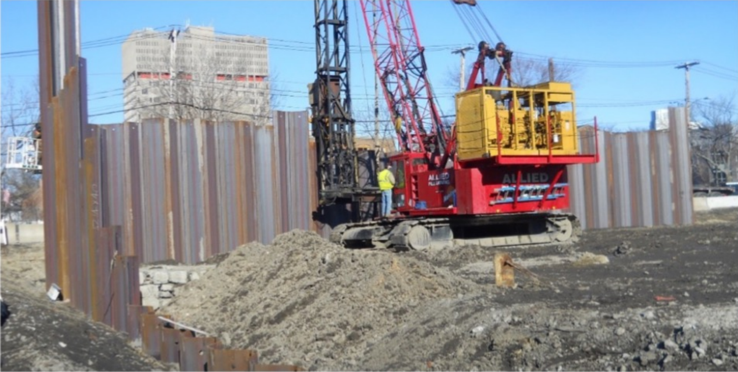
Sheet Pile Vibratory Head
