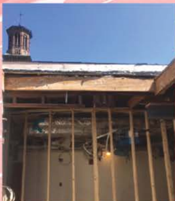
#5 St. Paul's $2.3MM in construction completed and 8,678 construction hours worked in 2020!
