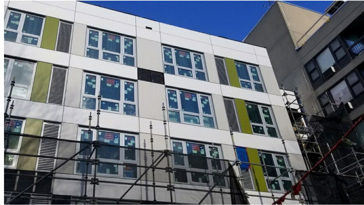
Burns Apartments part-way through construction
