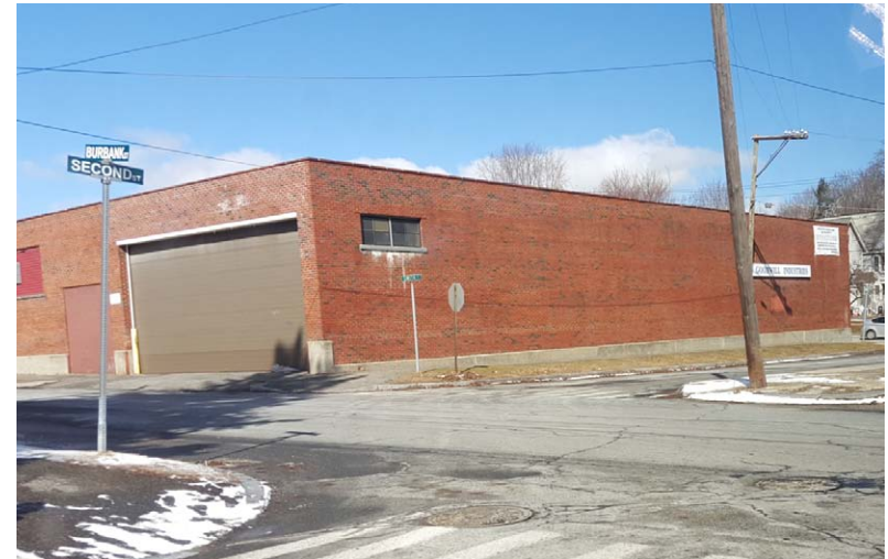
The Goodwill Building could improve its street frontage to interact with the street more
