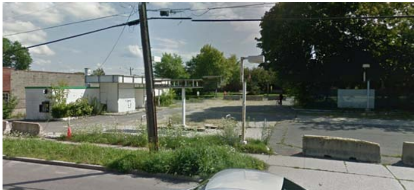
The Hess Property sits vacant and overgrown.
