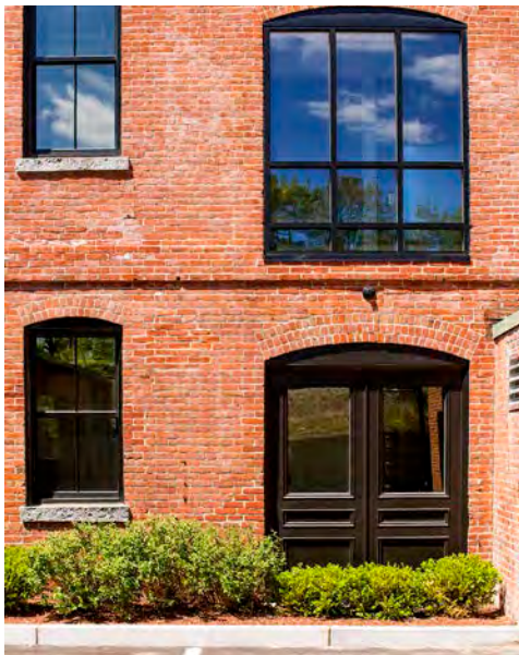
Top: Overview of building from back Middle: Model Unit Below: Detail
