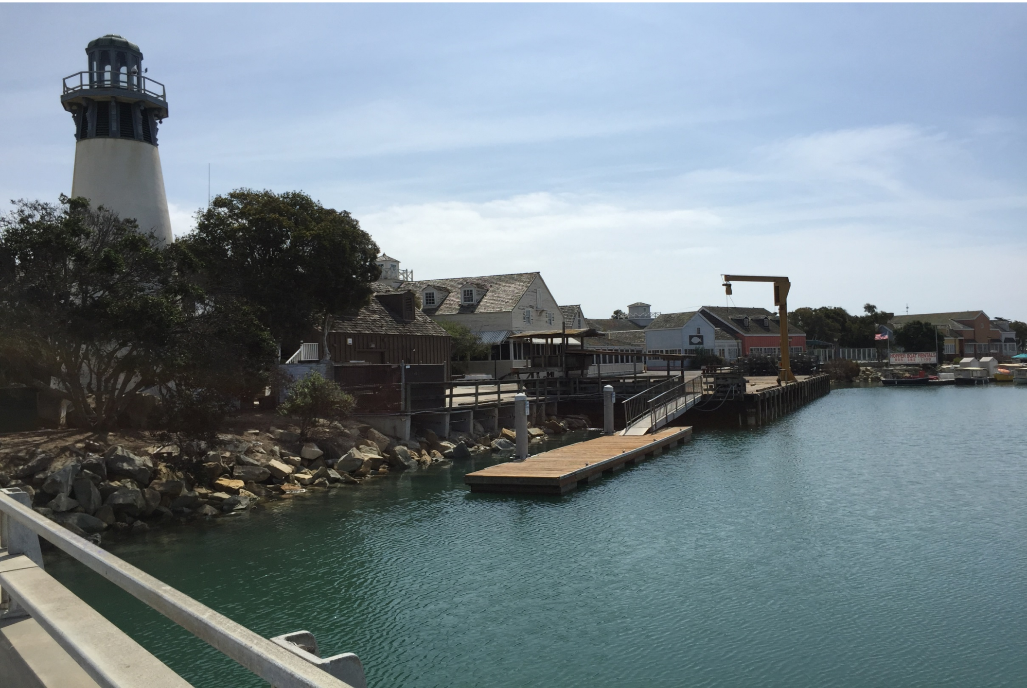
Channel Islands Blvd @ Bridge "Before"
