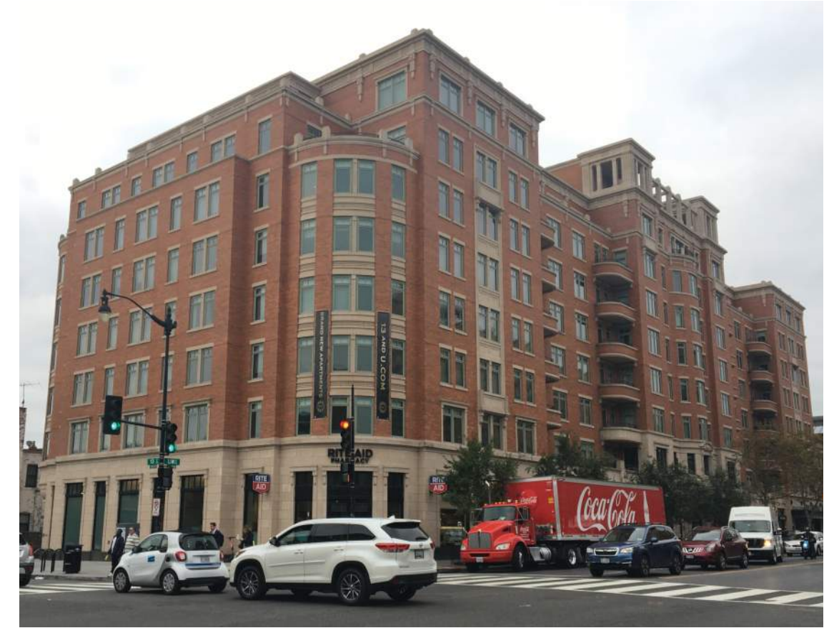
3. 13 | U Building - U Street, NW
