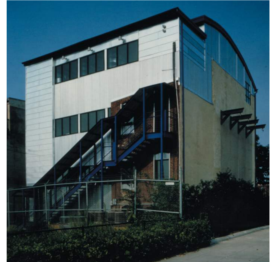
Rear of Townhomes Following Renovations
