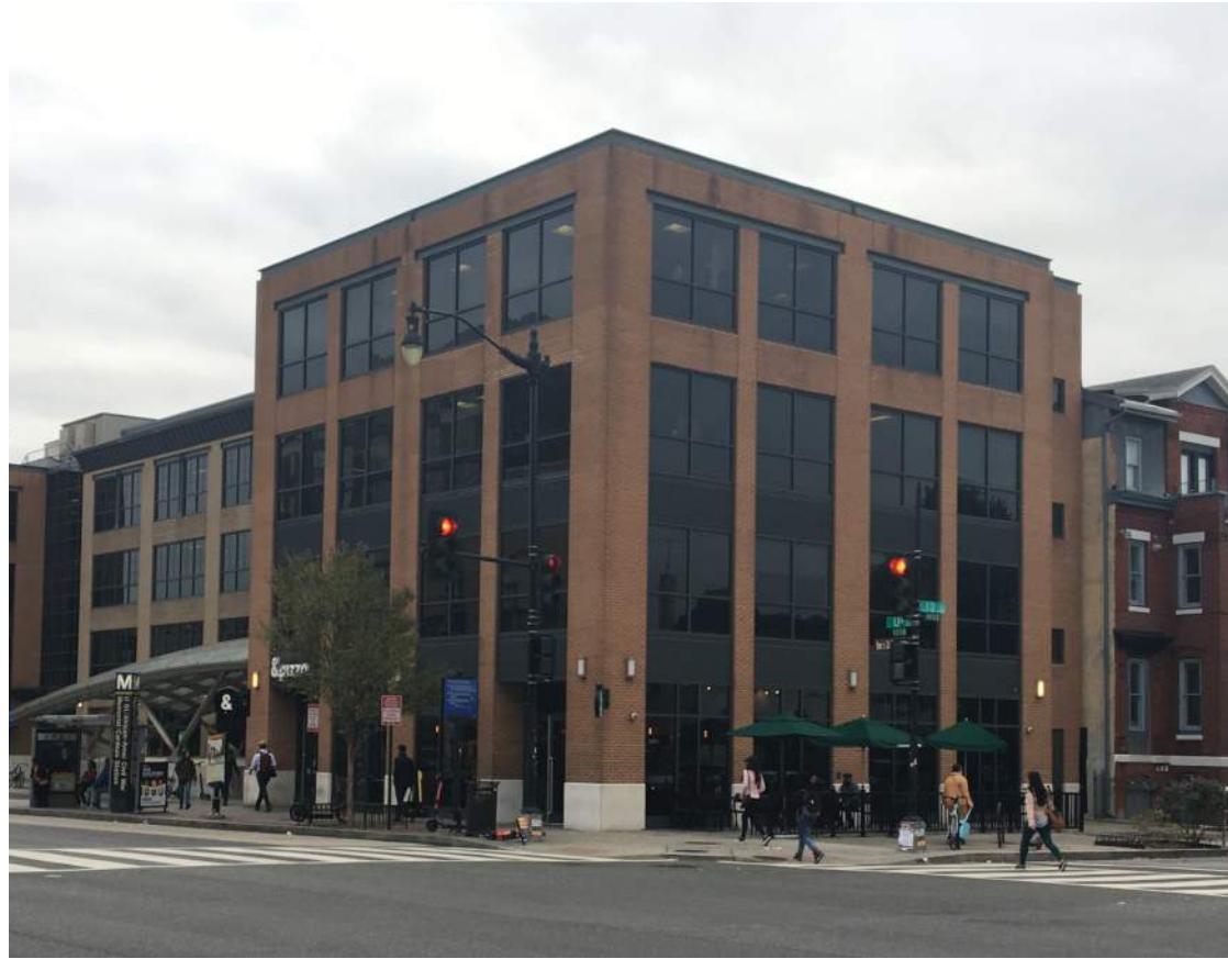
1. Existing Building North & West Facade - U Street, NW
