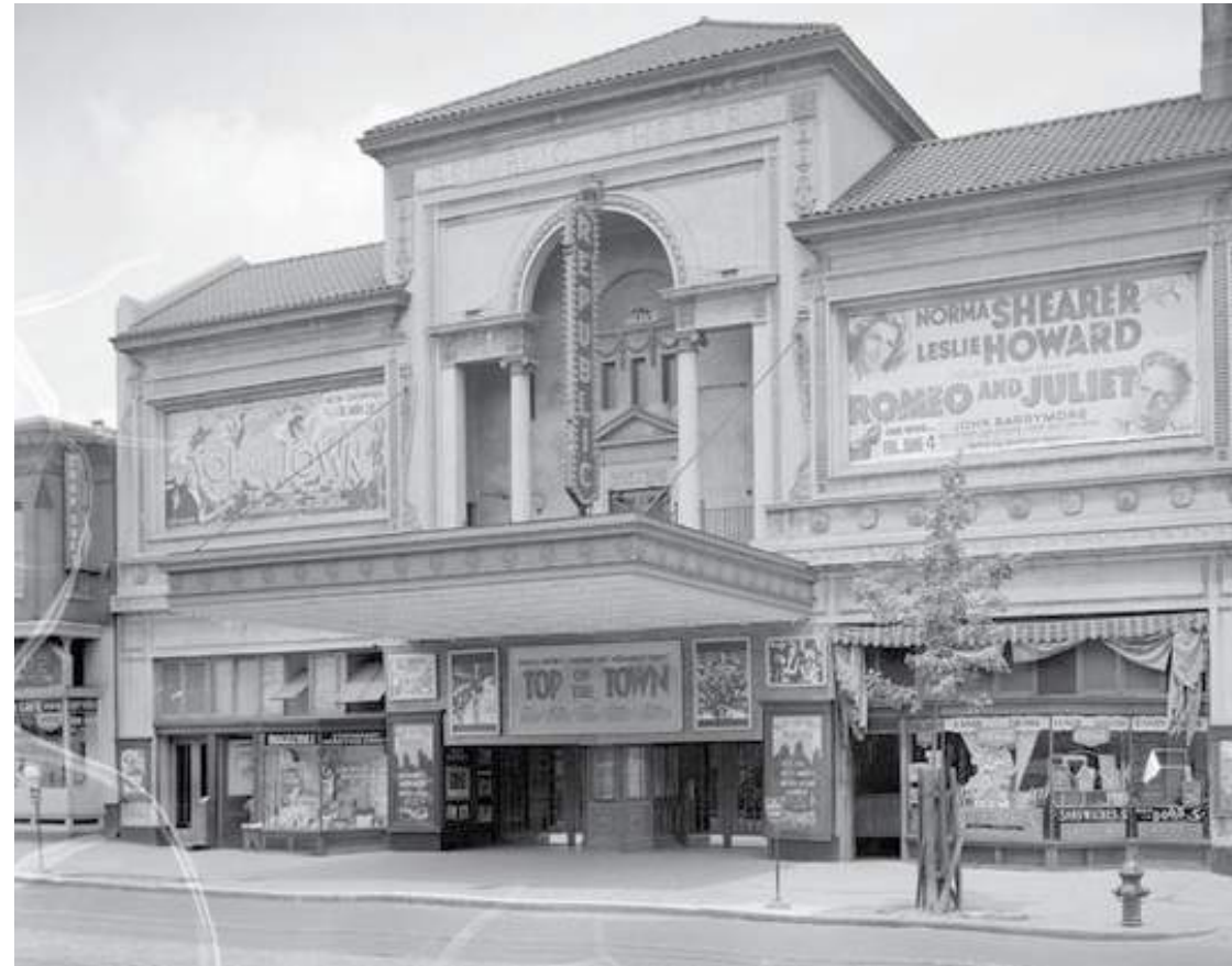
1. Republic Theater - U Street, NW (Demolished)
