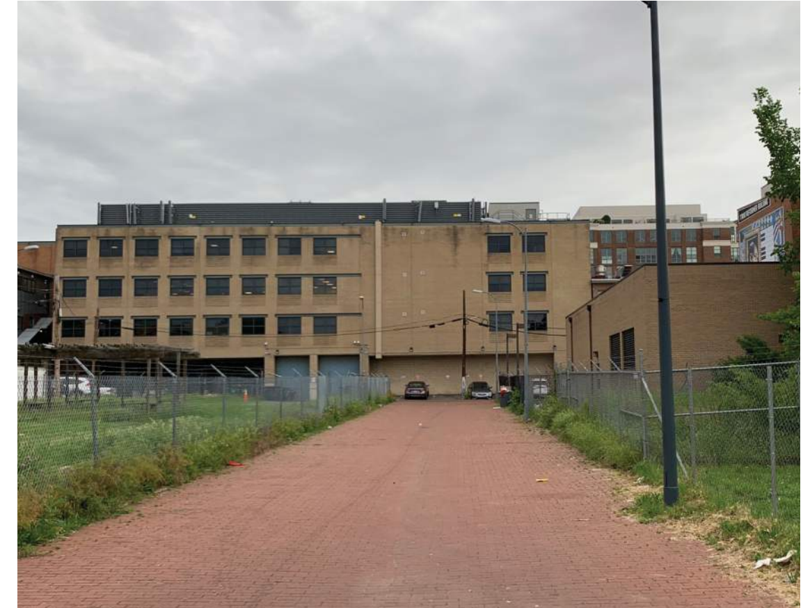
3. Existing Building South Facade - Temperance Ave, NW
