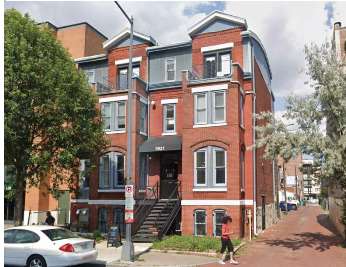
2. Existing Townhouses - 13th Street, NW
