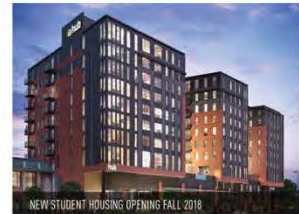
⑤ HUB on Campus: 11-stories, under construction, 1800 SF Retail 289 DU, 599 beds.
