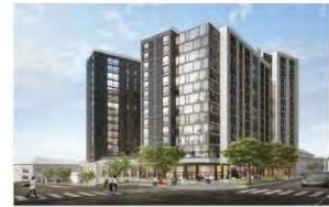
④ Rise at Chauncey: 16 Story, under construction, 300 DU, 675 beds.
