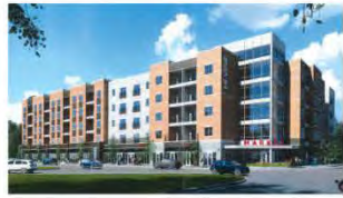
① HI Vine: 5 story, under construction, 12,580 SF Retail, 73 Apts, 117 Beds.
