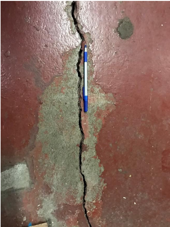
Photo 18. Maintenance Building. Concrete cracking in second floor slab.
