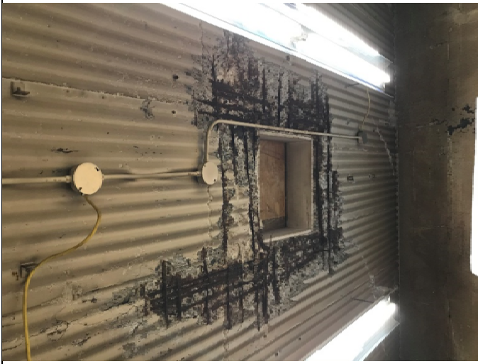
Photo 9 – Roof Slab Corrosion Deterioration
