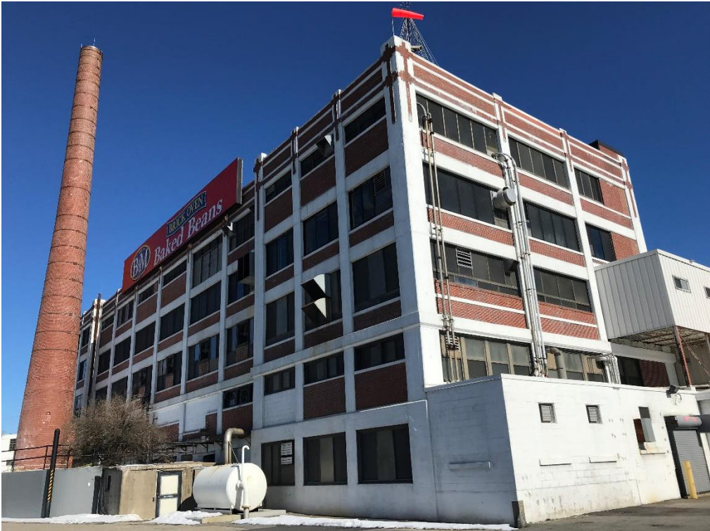
Photo 2. Main Factory Building. Exterior concrete surfaces have been recently repaired.
