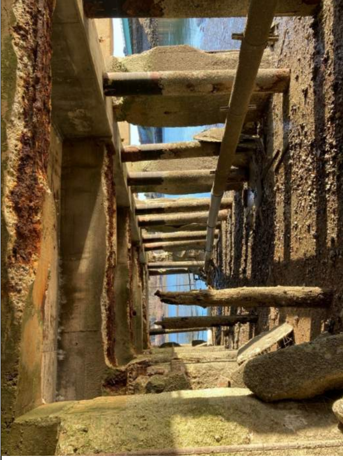
Photo 1 – First Floor Beam Corrosion Deterioration
