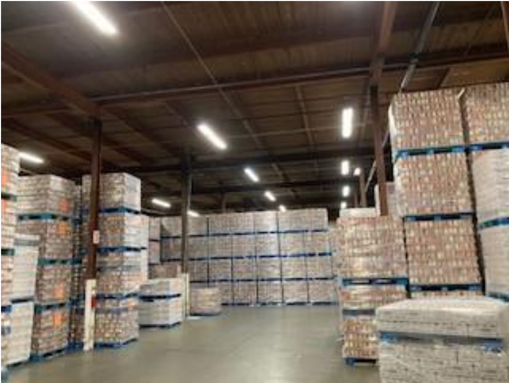
Photo 26. Warehouse No. 2. Similar to Warehouse No. 5, the one story steel framed building is in excellent structural condition with short term value as incubator or maker space.
