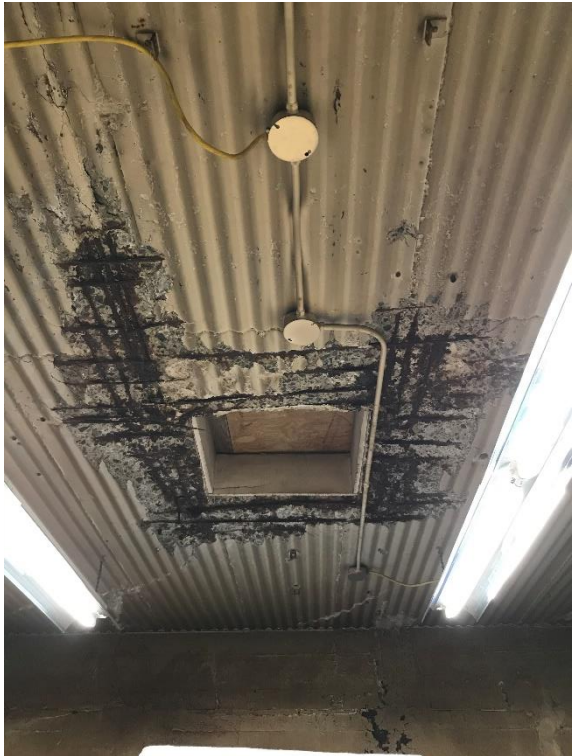
Photo 14. Maintenance Building. Concrete deterioration and reinforcing steel corrosion in roof slab.
