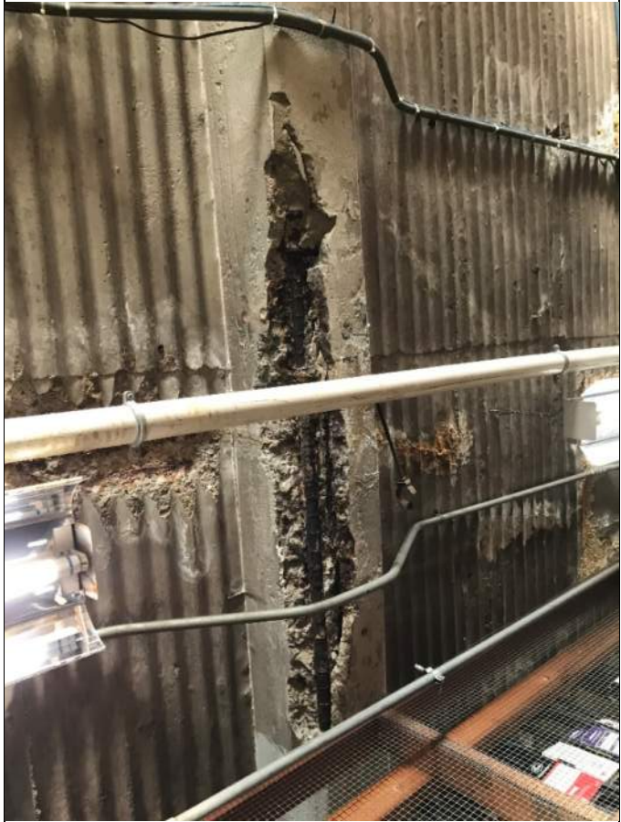
Photo 7 – Second Floor Slab and Beam Corrosion Deterioration
