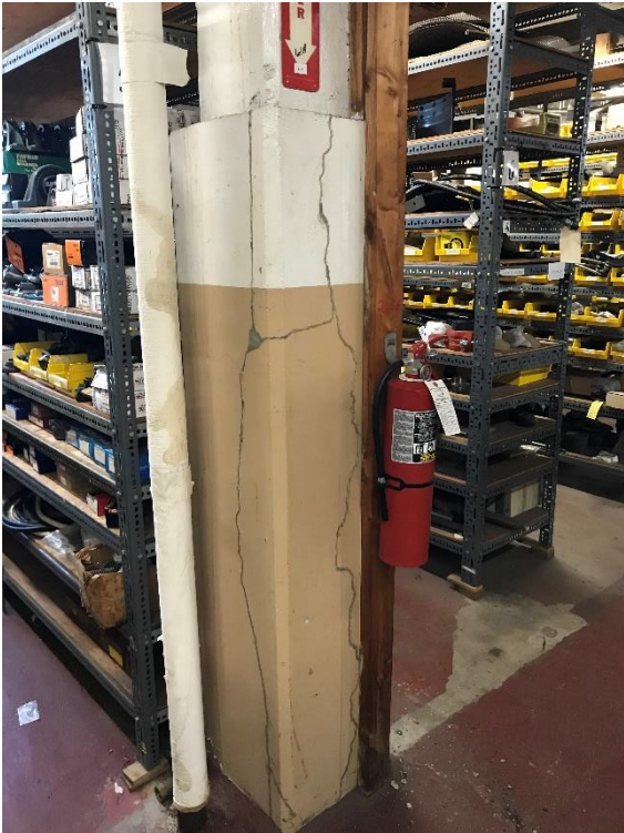
Photo 17. Maintenance Building. Concrete cracking in second floor column.
