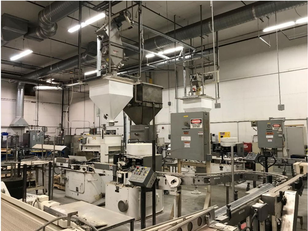
Photo 27. Spice Manufacturing Building. The circa 1980's steel framed building has large column gird and 22' high ceilings. The building is in excellent structural condition and has short term value as large meeting or incubator space.
