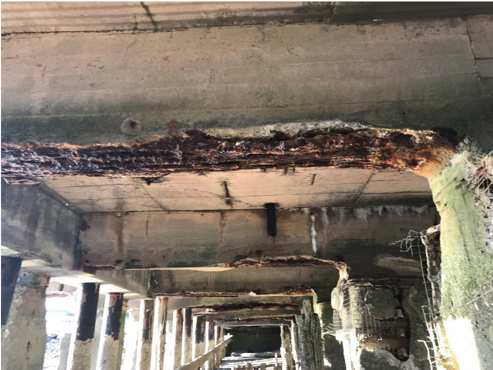
Photo 10. Maintenance Building. Concrete deterioration and reinforcing steel corrosion in the girders and piers.
