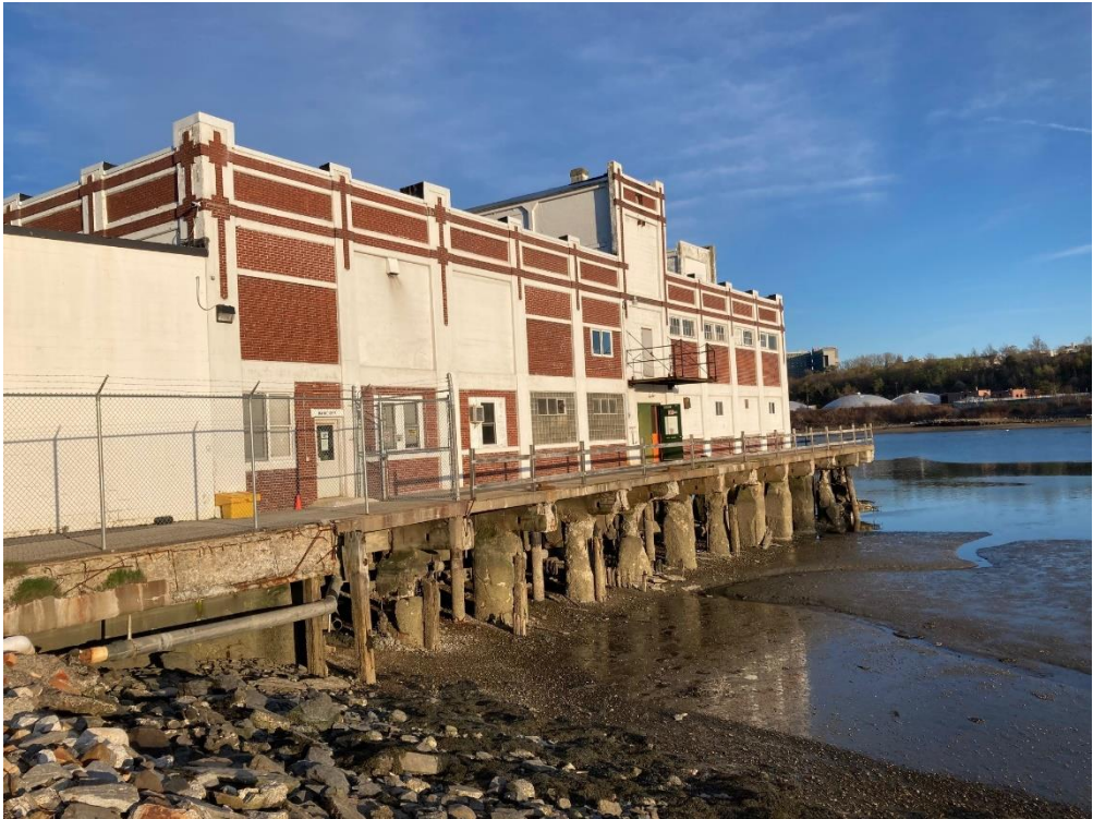
Photo 7. Maintenance Building on the Wharf (Former Cod-Fish Building). Constructed circa 1913.
