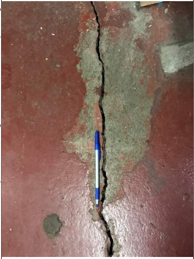
Photo 8 – Second Floor Slab Cracking
