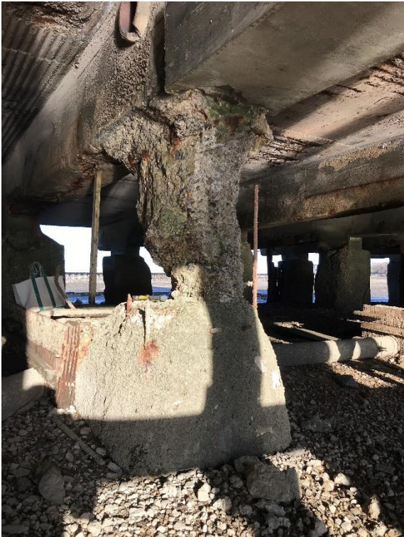
Photo 12. Maintenance Building. Deterioration has reduced the size of a concrete pier from 48" by 48" to 10" by 10". The owner was alerted of safety concerns.
