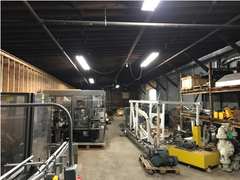
Photo 22. Warehouse No. 28. Low bay wood framed structure with newly framed exterior wall could provide ancillary space to gymnasium or fitness center located in attached Warehouse No. 4.
