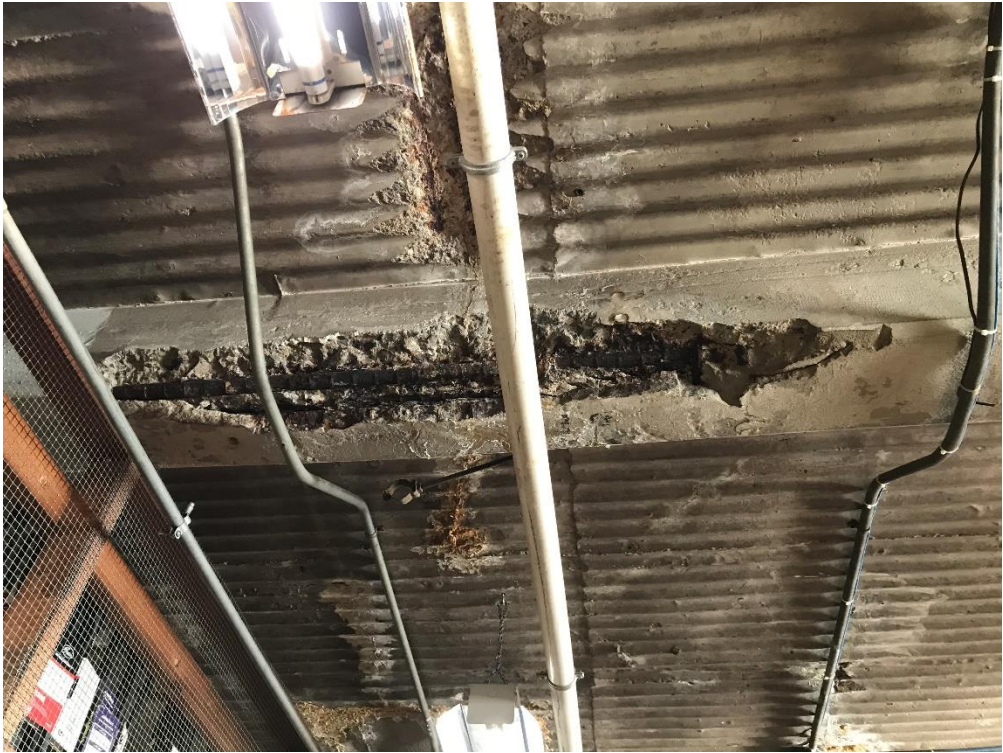
Photo 13. Maintenance Building. Concrete deterioration and reinforcing steel corrosion in roof beam.
