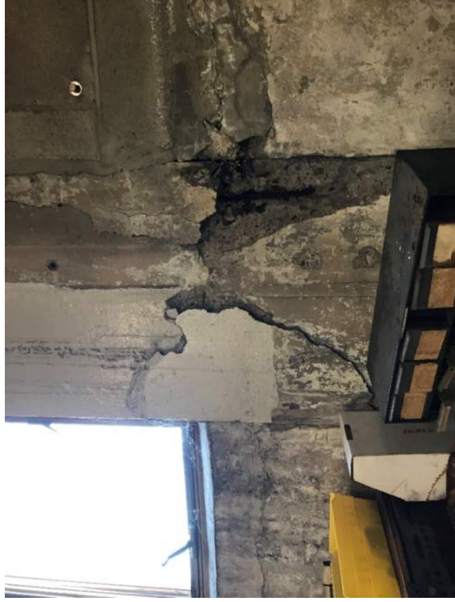
Photo 10 – Exterior Roof Column Corrosion Deterioration
