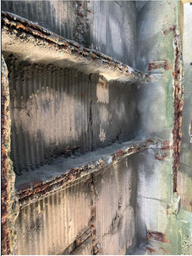
Photo 3 – First Floor Slab Corrosion Deterioration
