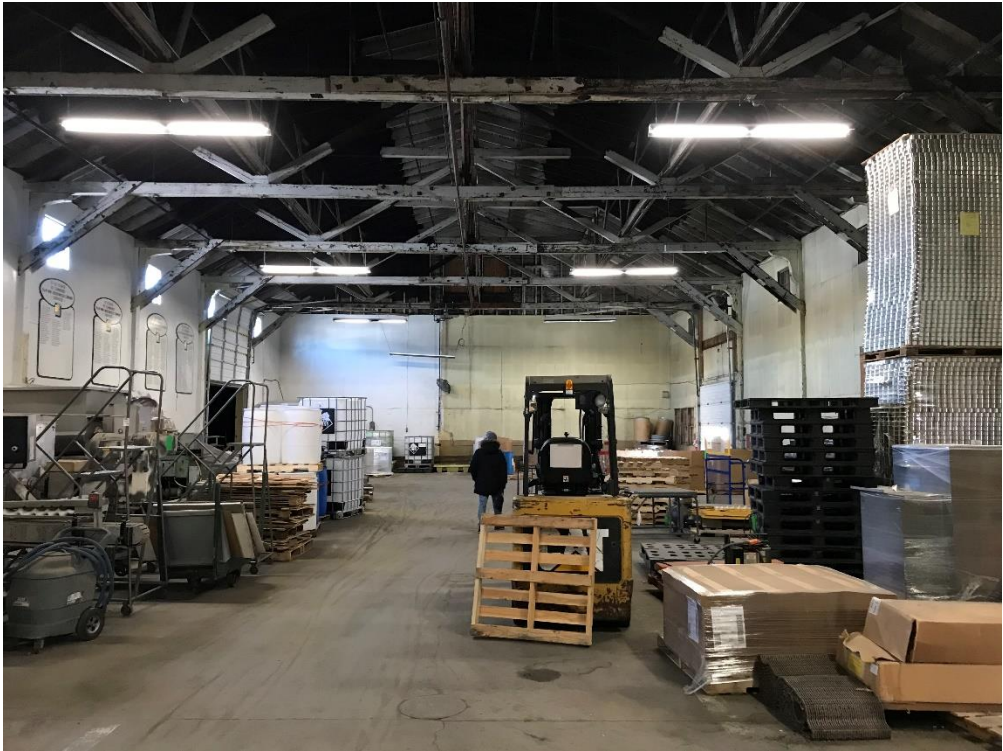
Photo 21. Warehouse No. 4 (White Barn). 50' wide by 130' long column free space with potential reuse as gymnasium or fitness center.
