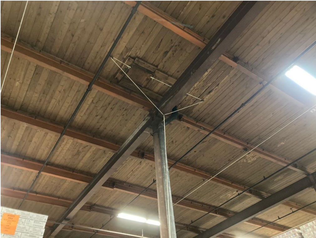
Photo 24. Warehouse No. 5. Steel framing is laid out on 24' by 25' column gird with 20' high exposed wood roof deck ceilings. The building is in excellent structural condition.
