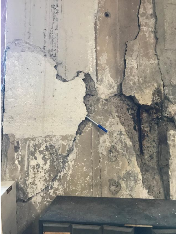
Photo 15. Maintenance Building. (Before removing spall) Concrete cracking in second floor column.
