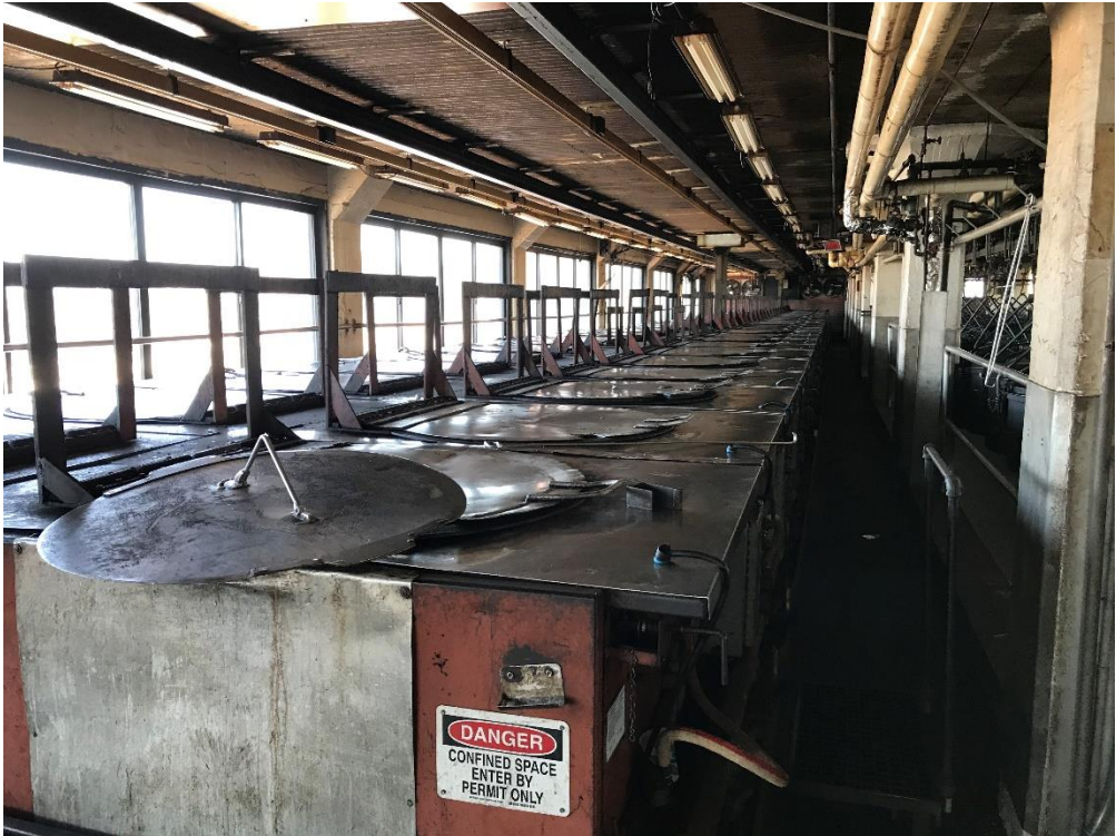
Photo 3. Main Factory Building. Heavy bean ovens located on the fourth floor.
