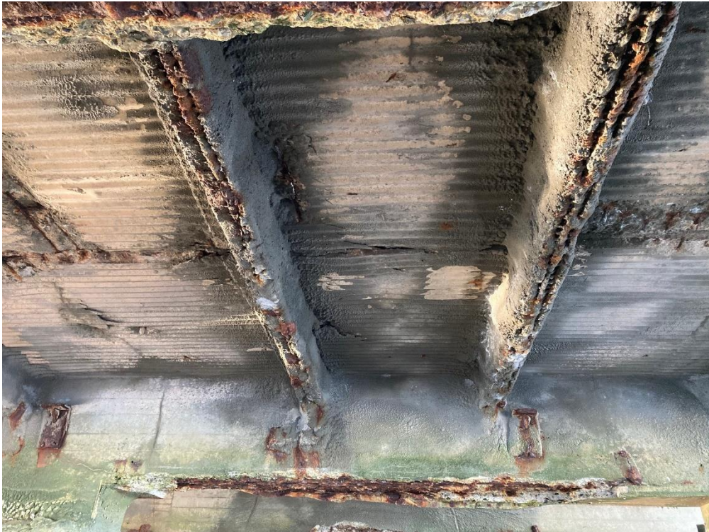
Photo 11. Maintenance Building. Deteriorated concrete floor slab and girders under the wharf.
