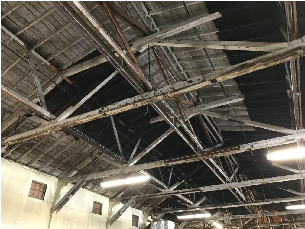
Photo 20. Warehouse No. 4. High bay wood roof trusses.
