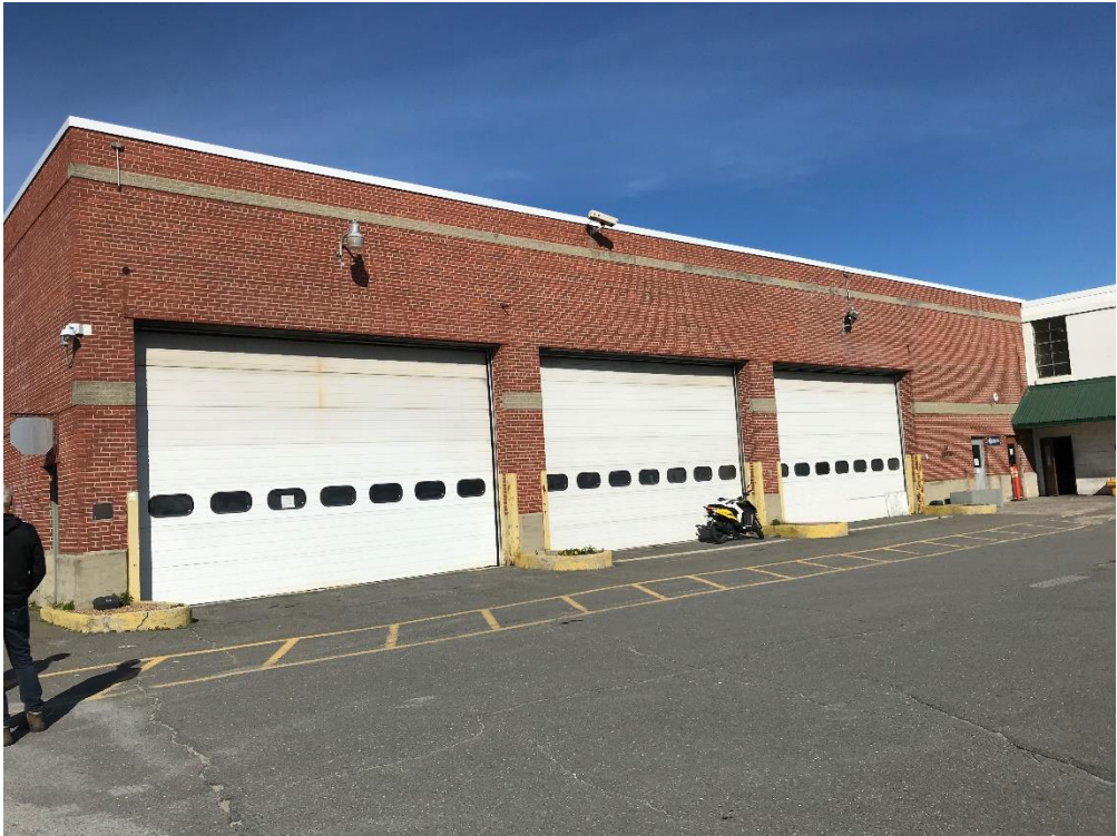
Photo 23. Warehouse No 5. Circa 1950's one story steel framed building with exterior brick veneer and CMU walls.
