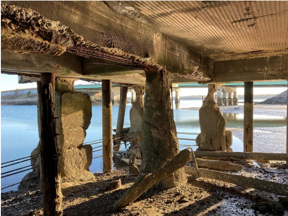
Photo 9. Maintenance Building. Deteriorated concrete girders and pier under the wharf.
