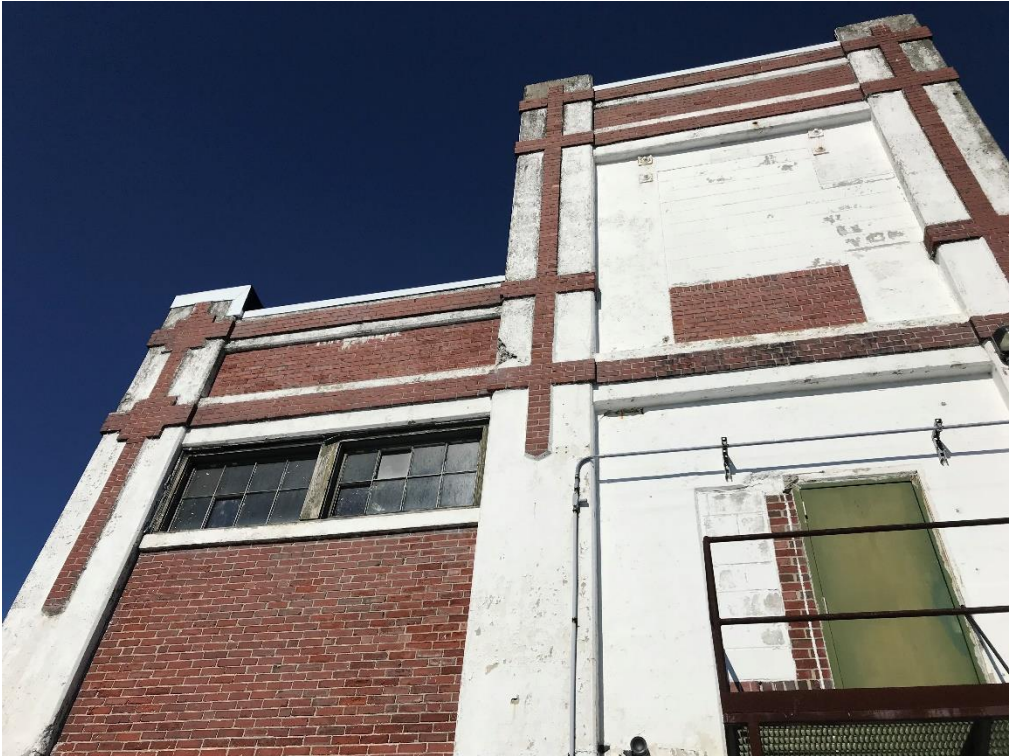
Photo 8. Maintenance Building. Exterior building condition.
