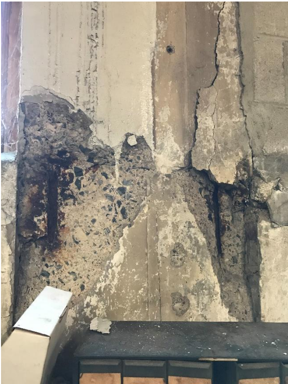
Photo 16. Maintenance Building. (After removing spall) Corroding reinforcing steel caused column spall.
