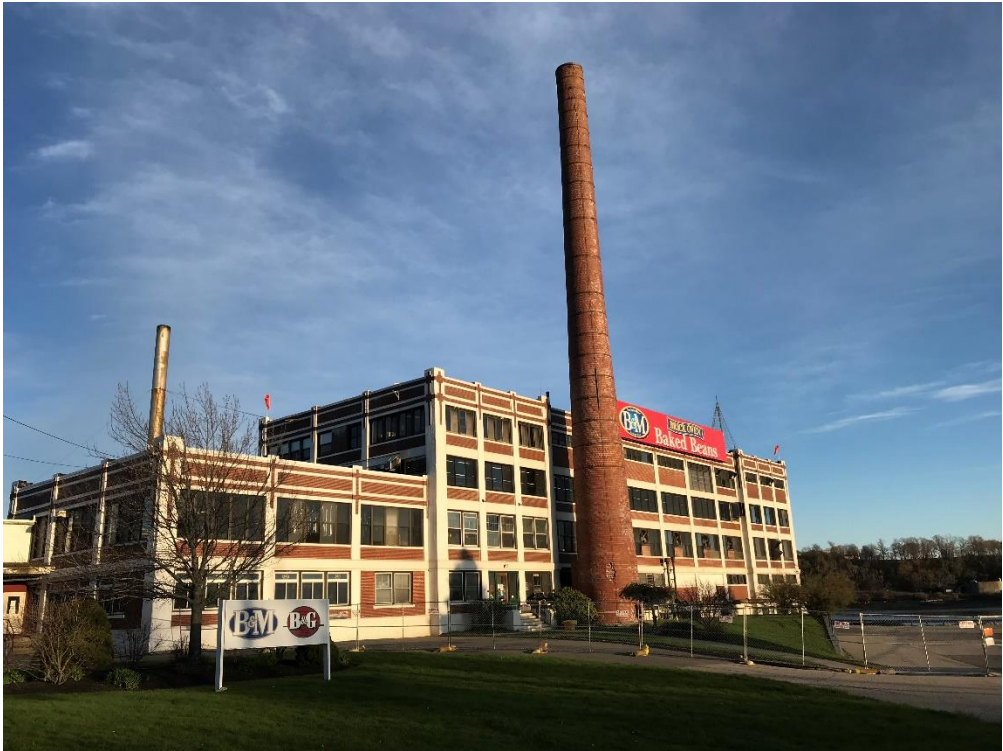
Photo 1. Main Factory Building. Constructed circa 1912, the building has long term value as housing, hospitality or office space.
