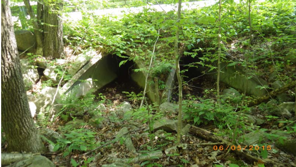
Photo 1 – Culvert under MBTA Road, Outlet from Eastern Wetland
