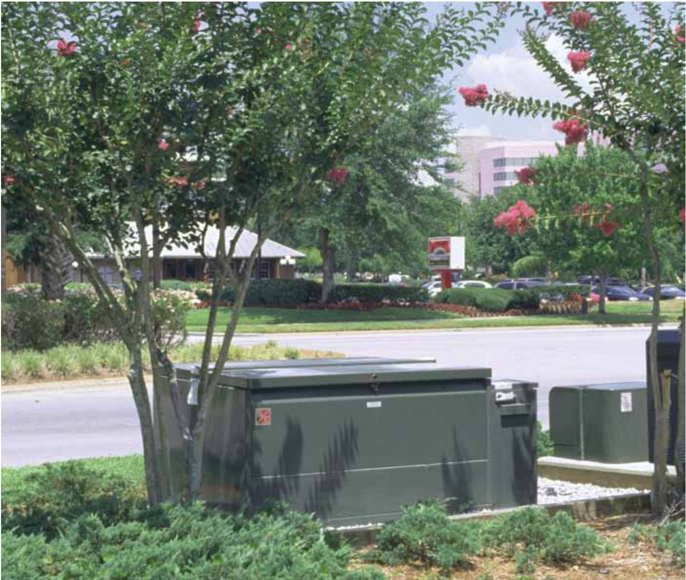
Remote Supervisory Pad-Mounted Style Vista UDS installation.
