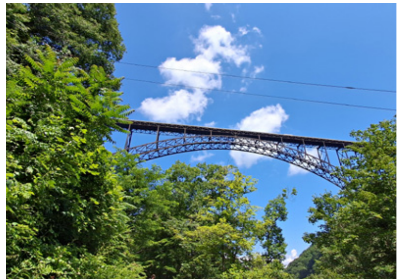
View of New River Bridge from below
