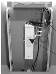
Power supply cables Control unit
