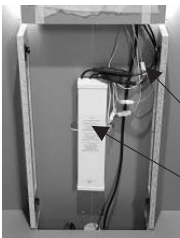
Power supply cables Control unit
