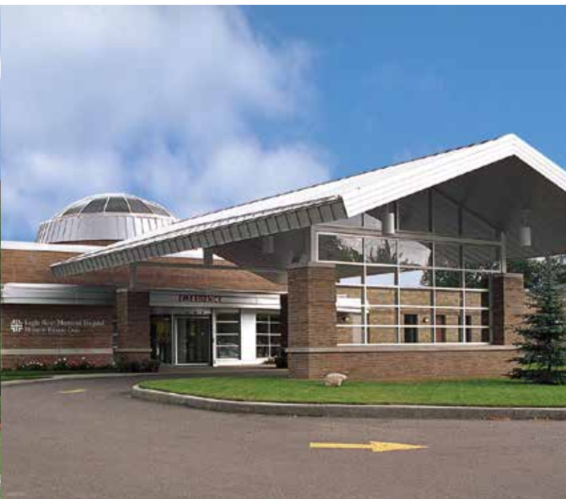
Ascension Eagle River Hospital, Eagle River, WI
