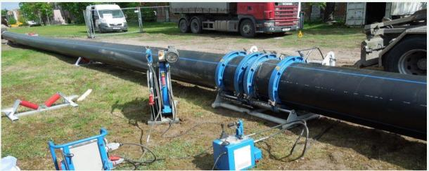
Figure 1. HDPE pressure pipes installation process stage
