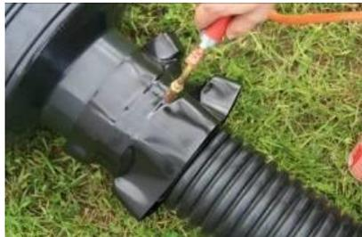
*EN The shrinking is carried out using a soft flame operated from a gas cartridge or a hot air gun at medium temperature. First, shrink an approx. 4 cm broad area where the casing pipe enters/exits the connected half shells. Once shrunk work your way towards the casing pipe, then connected half shell element.*
