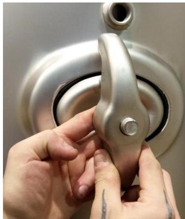
5. Centre the seal and handhole before tightening.
