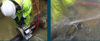
For greater cutting depth there is an option to purhcase 180 mm blades. Available models: **Diamond X 180** – cast iron, **Cermet 180** – stainless steel, carbon steel, **ALU 180** – plastics and aluminium.
